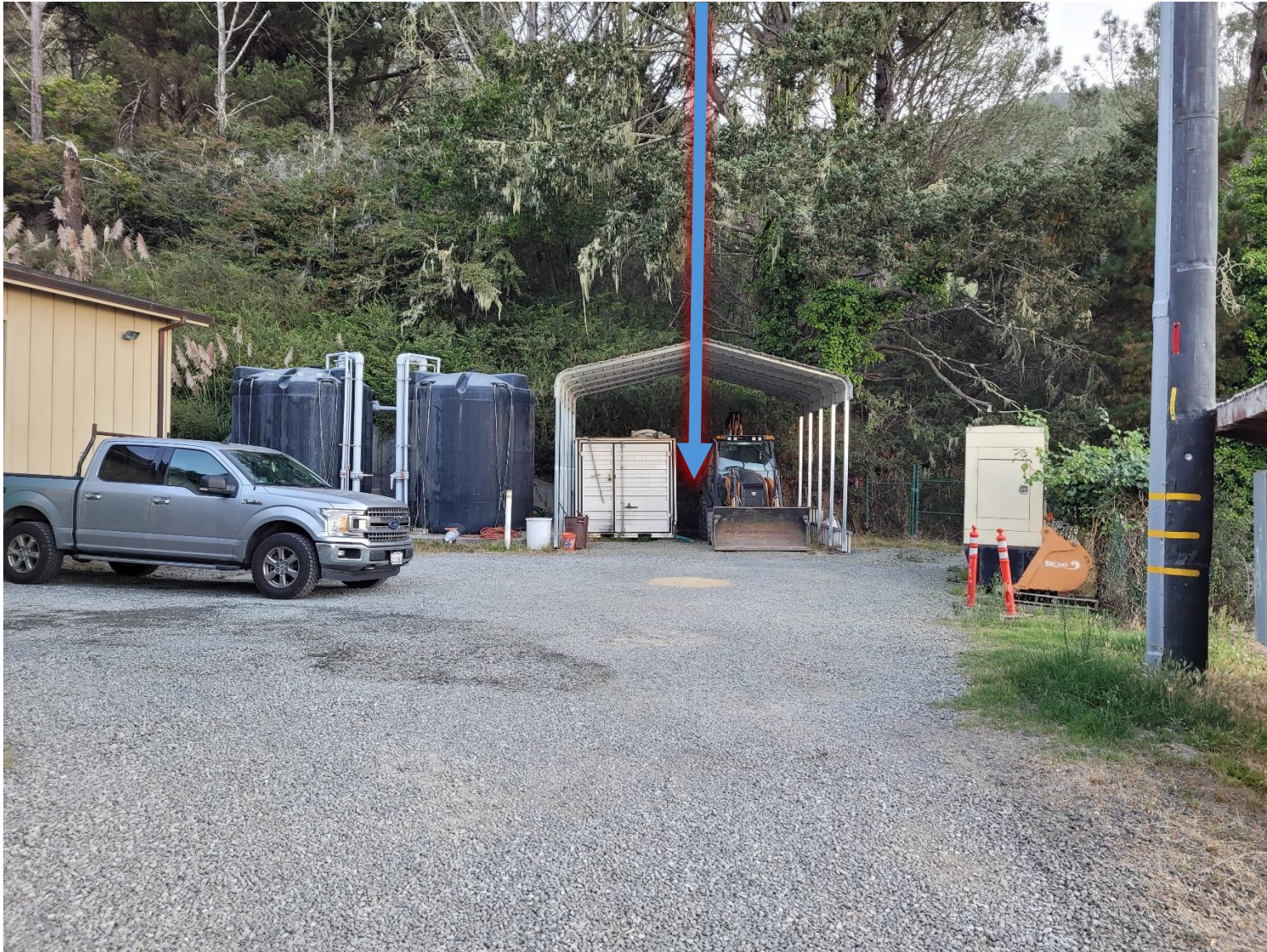
Photo 1: Existing Water Treatment Plant building.
