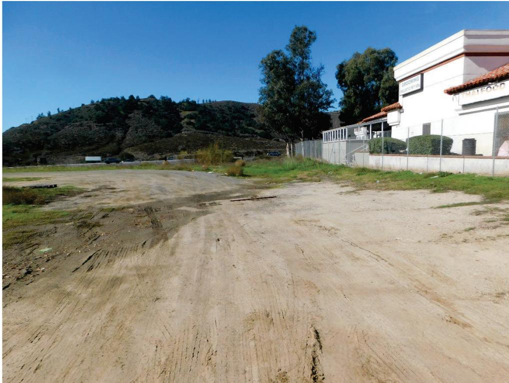
**Photograph 12:** Evidence of sheet flow from the middle of the project site to the northwest corner of the project site. The sheet flow of water during and immediately following storm events across this portion of the site follows onsite topography that was created when the site was graded.
