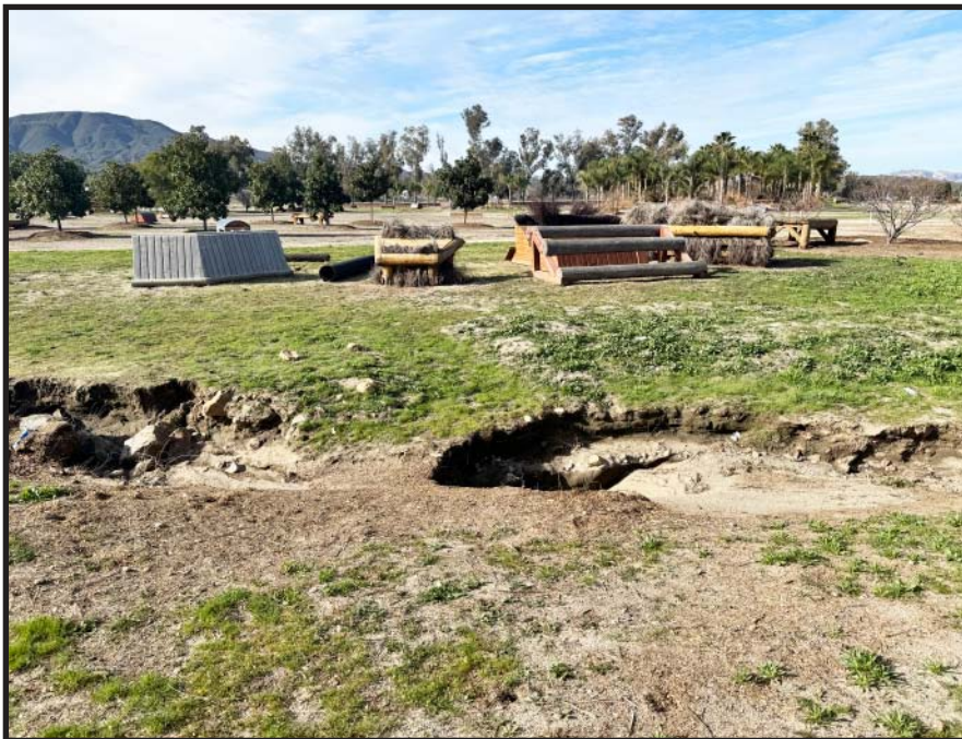
PHOTOGRAPH 16 - Southwest view of equestrian facilities and ephemeral drainage which bisects the northern region of Project Site.
