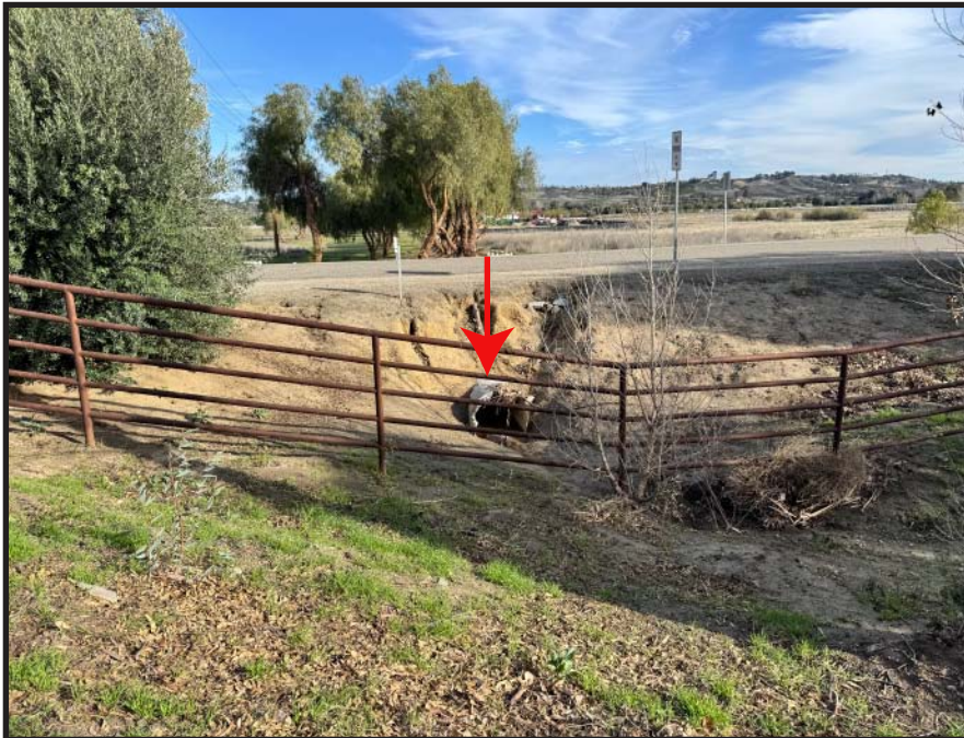
PHOTOGRAPH 6 - Northward view of culvert which extends north from the Project Site to Temecula Creek.
