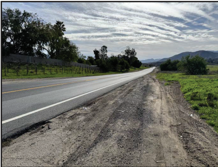
PHOTOGRAPH 22 - Southeast view of offsite impact area from the intersection of SR79 and Los Caballos Road.
