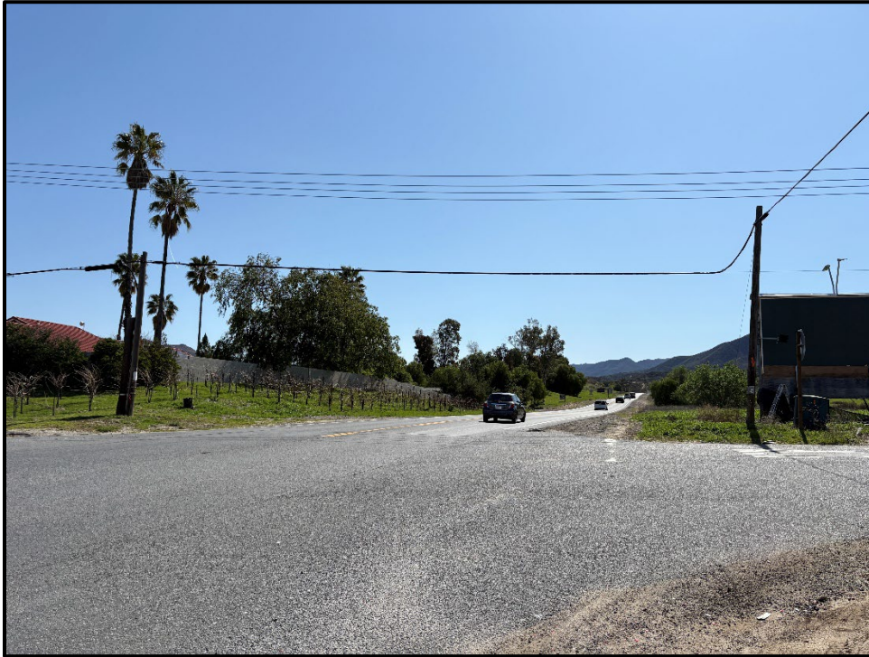
Plate 4.2-4: Overview of the off-site improvement area of the project near the intersection of SR 79 and Los Caballos Road, facing southeast.
