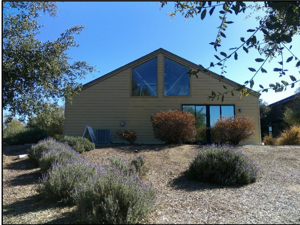
Plate 4.2-8: Overview of the historic building, constructed between 1967 and 1976 within the Galway Downs property (Temp-1), which currently functions as a sales office, facing northeast.
