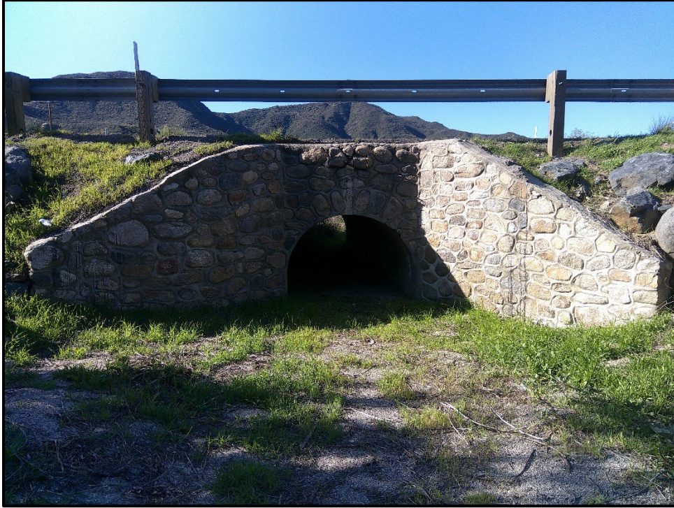
Plate 4.2–10: Overview of the arched bridge culvert near the intersection of Pauba Road and SR 79 (Temp-2), facing southwest.
