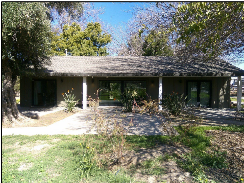
Plate 4.2-9: Overview of the historic building, constructed between 1967 and 1976 within the Galway Downs property (Temp-1), facing northwest.
