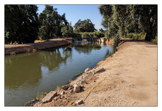
Figure 5. The Main Intake Canal within the St. Johns Siphon APE. Note the headwalls on either side and the trash rack at the center. View toward southeast.
