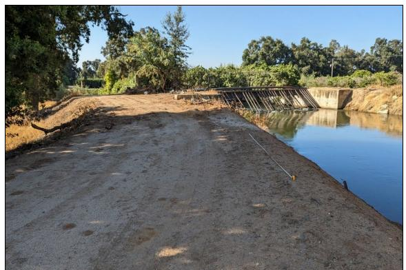
Figure 6. St. Johns River siphon APE, pictured in rear. Note the headwalls and trash rack. View toward southeast.
