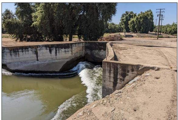
Figure 9. View of the Kaweah River siphon intake head walls and wing walls. View toward south.
