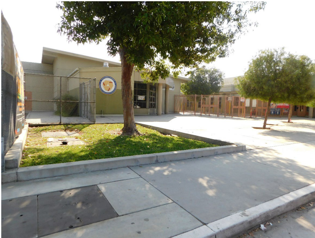
Photograph 6 From the western edge of the Tweedy Elementary School site, looking east.
