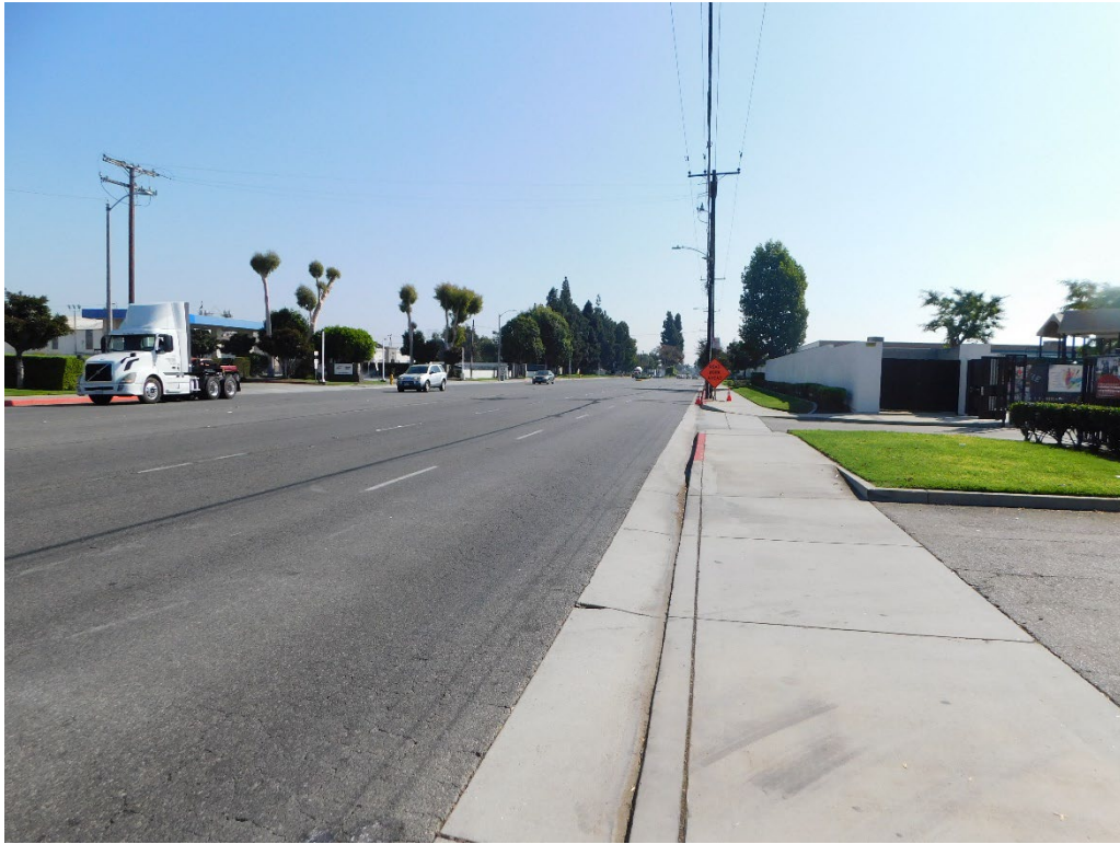
Photograph 9 From the northwestern corner of the Tanner Elementary School site, looking east along the proposed alignment.
