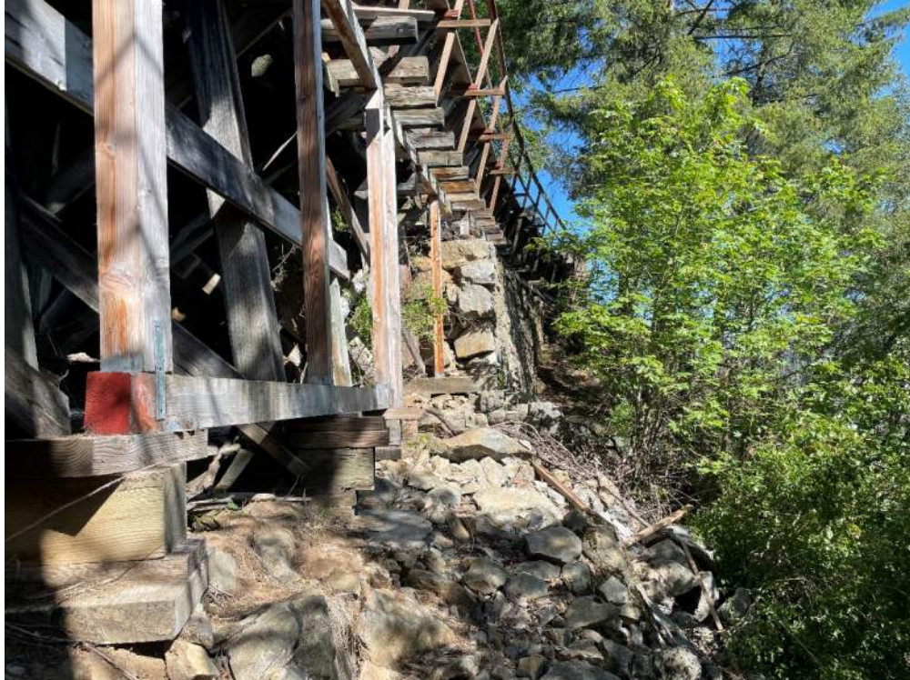
View of Flume 48 project site from below, facing west.
