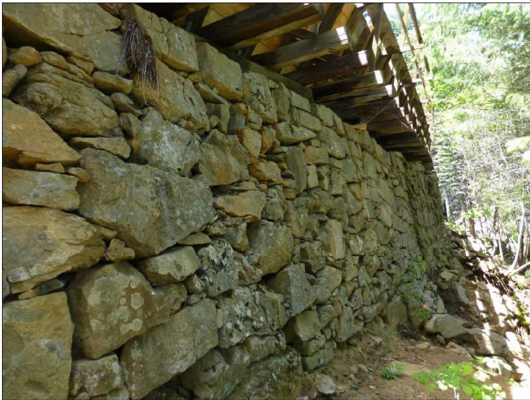
Photo 2: Flume 48 existing rock wall foundation
