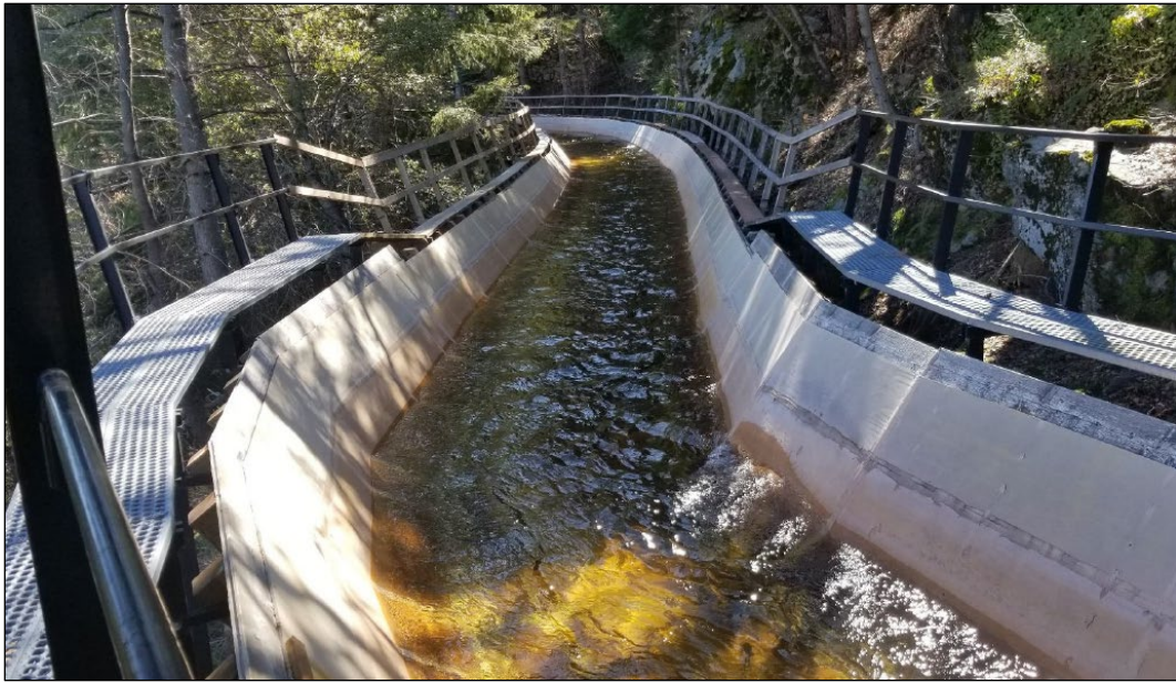
Photo 1: Section of Flume 48
