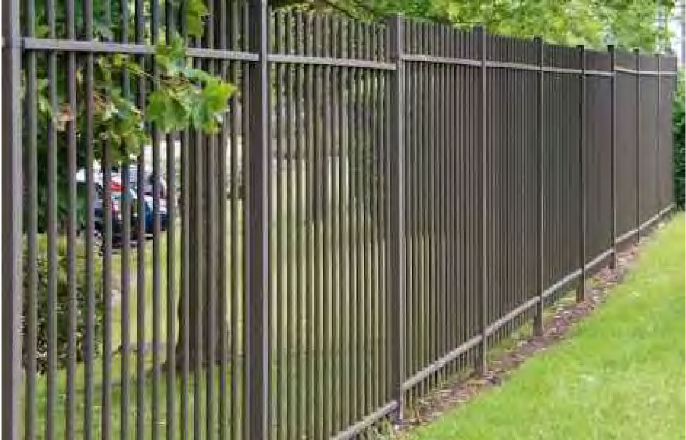
TUBULLAR STEEL PROPERTY FENCE
