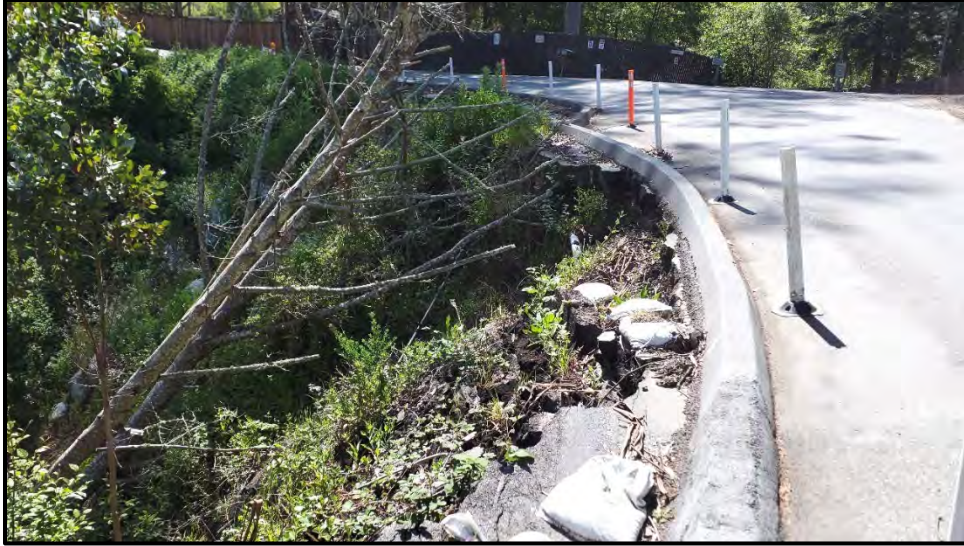
Photograph A-3. Slide along north shoulder of Higgins Canyon Road; view facing southeast. Photograph taken May 2, 2024.
