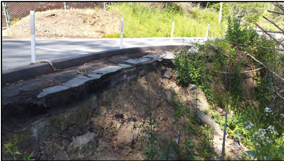
Photograph A-4. Slide along north shoulder of Higgins Canyon Road; view facing west. Photograph taken May 2, 2024.
