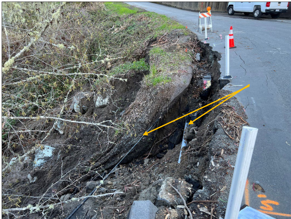
Photo 4: East-facing view of the slip-out area. Note the two exposed utility lines in the scarp area. The photo was taken on March 8 th , 2023.
