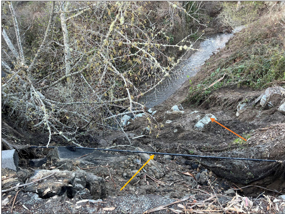
Photo 5: Northeast-facing view of the slip-out area. Note the exposed utility line (see yellow arrow). Also note exposed riprap in slope fill (orange arrow). The photo was taken on March 8 th , 2023.
