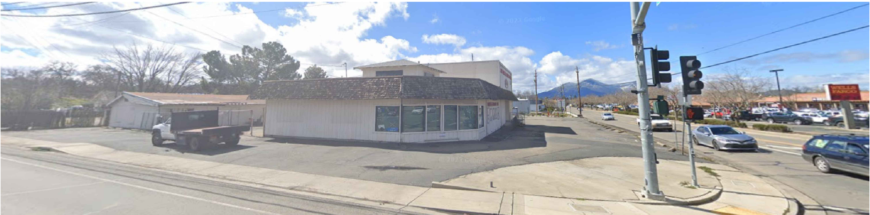
CORNER VIEW @ OLD HIWAY 53 AND OLYMPIC DR.
