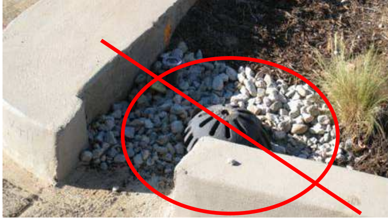
Figure 6: Incorrect Placement of an Overflow Inlet.
