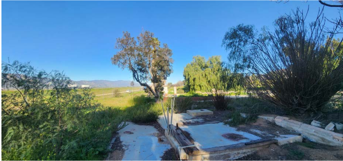
Photograph 3: View of a foundation from a previous development in the western portion of the study area, facing north.
