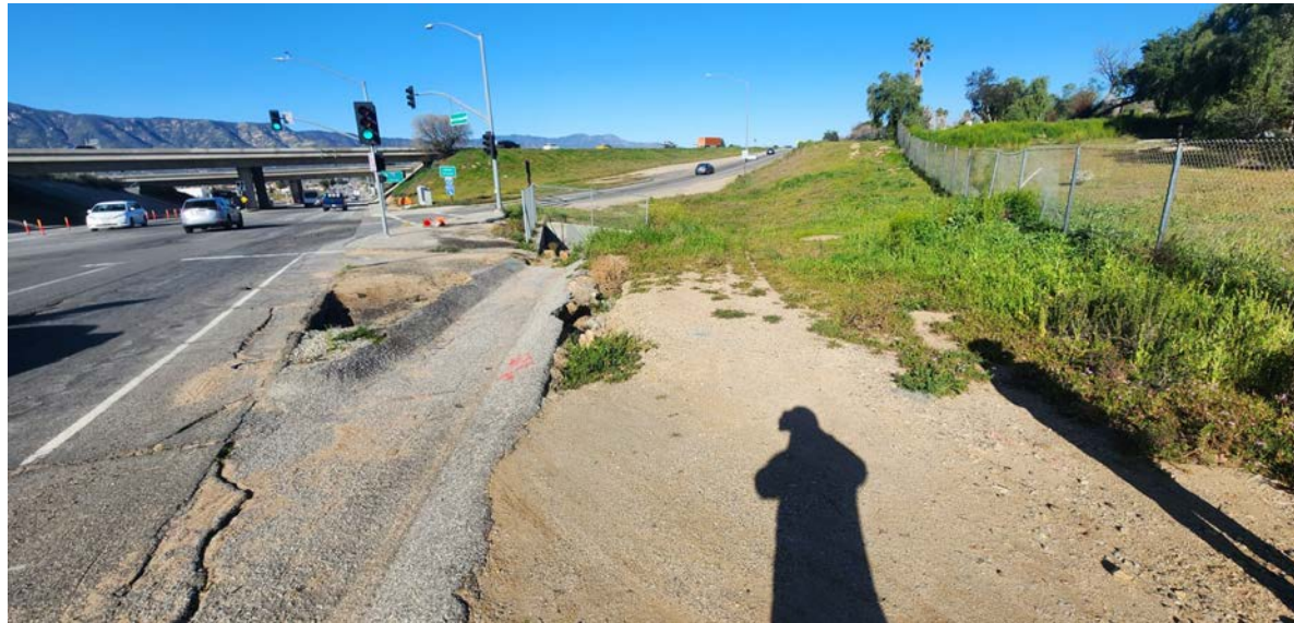
Photograph 6: View of the ribbon gutter and culvert in the southwest portion of the study area, on the north side of Bundy Canyon Road.
