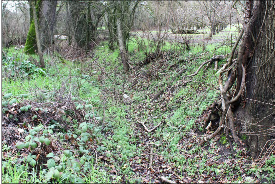
Photograph 2: North end of drainage ditch, just south of where it empties into natural slough; facing southwest, February 8, 2024.
