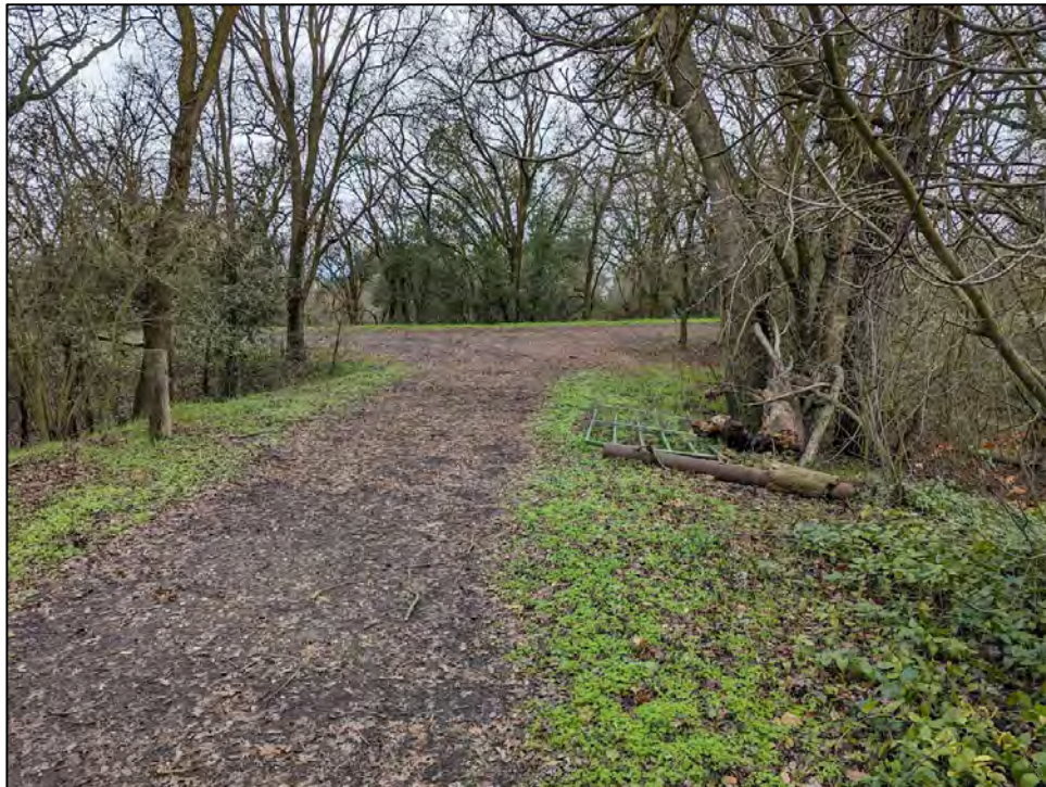
Photograph 7: West end of Feature D, RD 554 Levee, showing junction with Railroad Embankment; facing west, February 8, 2024.
