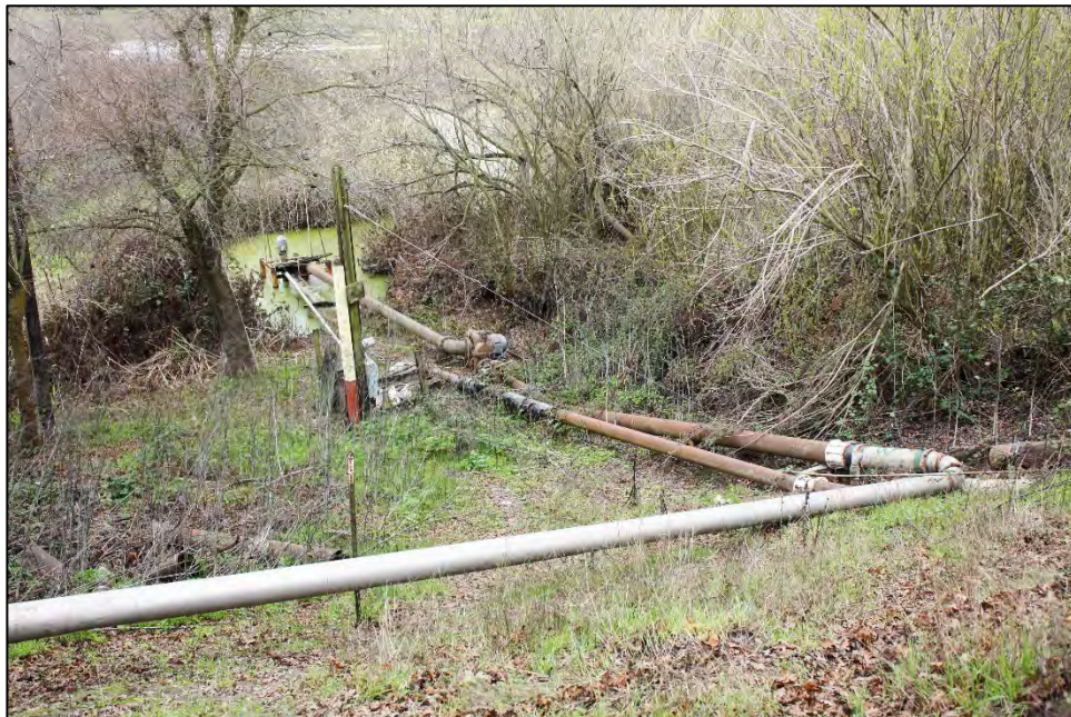
Photograph 15: Pipelines extending from pump in drainage ditch on southwest side of levee. The pumping station is outside of state Property boundaries. The older rust-colored pipeline passes through levee beneath crown. The newer line crossing diagonally through photograph has been emplaced to bypass the older line; facing west, February 8, 2024.
