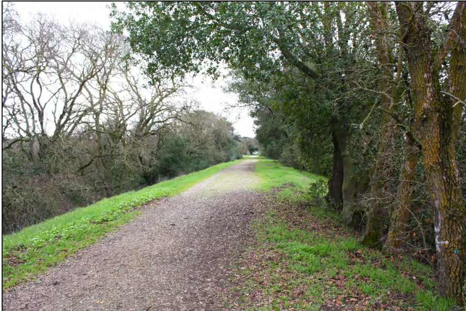
Photograph 10: Feature E, Railroad Embankment, approximately 1,000 feet north of south Property boundary; facing south, February 8, 2024.
