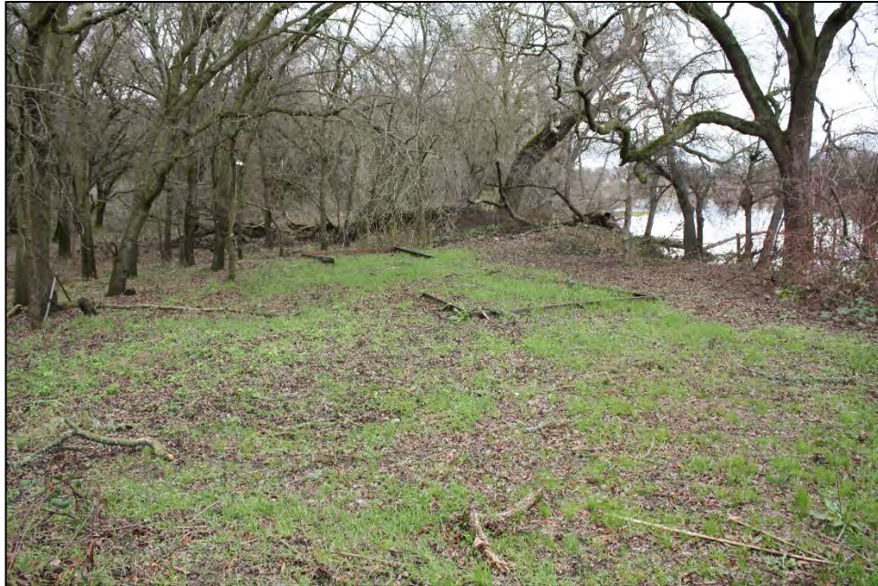
Photograph 16: Feature G, RD 551 Levee Berm, showing wide surface area with Meadows Slough to the south (left); facing southeast, February 8, 2024.
