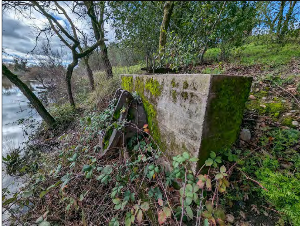
Photograph 6: East end of pipe, discharging into Railroad Cut Slough; facing south, February 8, 2024.
