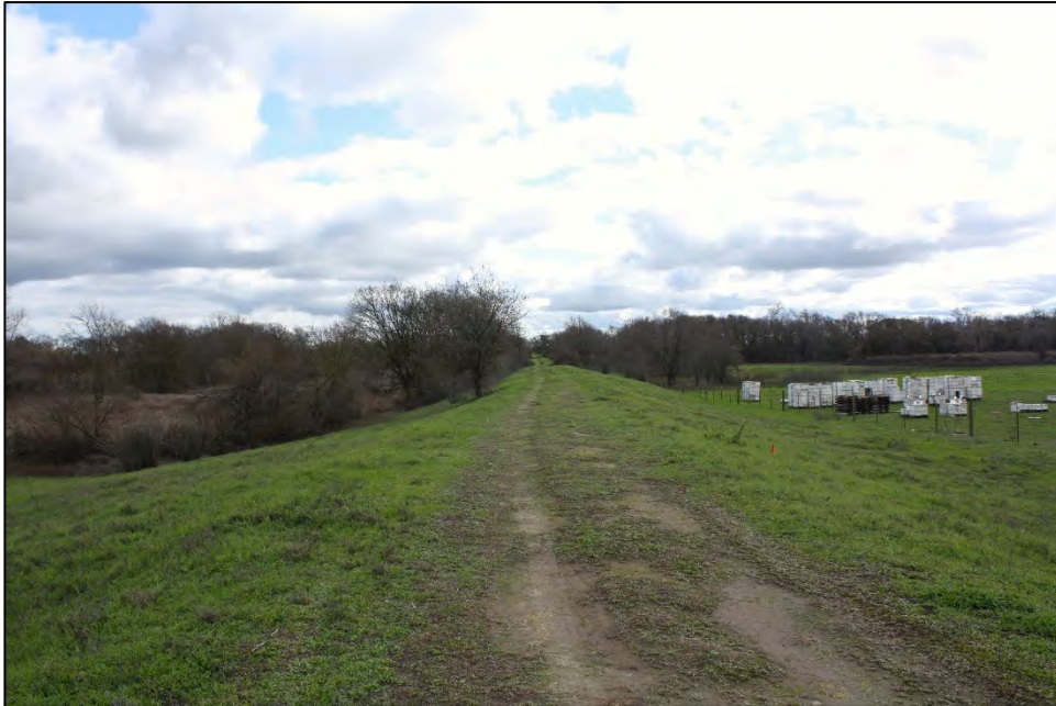
Photograph 12: The southeast segment of Feature F, Locke Levee, with private Locke Ranch to south (right) and seasonal pasture and wetlands to north (left); facing southeast, February 8, 2024.
