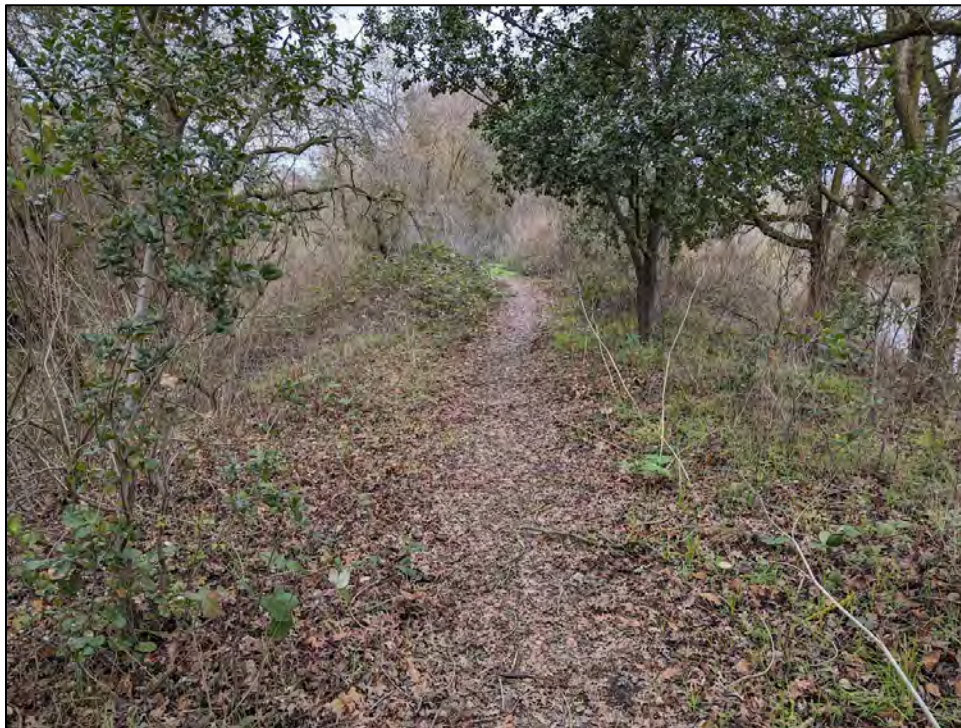
Photograph 13: The northwest segment of Locke Levee showing thick vegetation and narrow foot trail; facing northwest, February 8, 2024.
