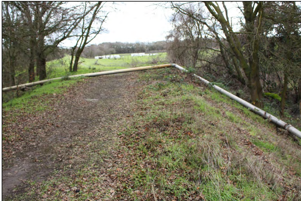
Photograph 14: Recent pipeline addition laid across crown of Locke Levee; facing southeast, February 8, 2024.
