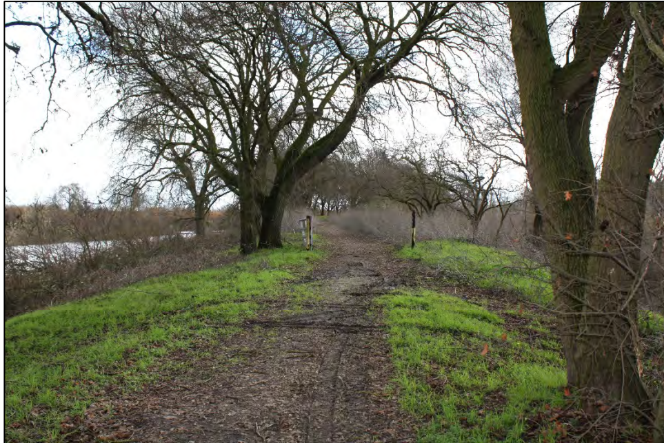
Photograph 8: East end of recorded segment of RD 554 Levee with the gate in mid-distance marking the Property boundary; facing east, February 8, 2024.
