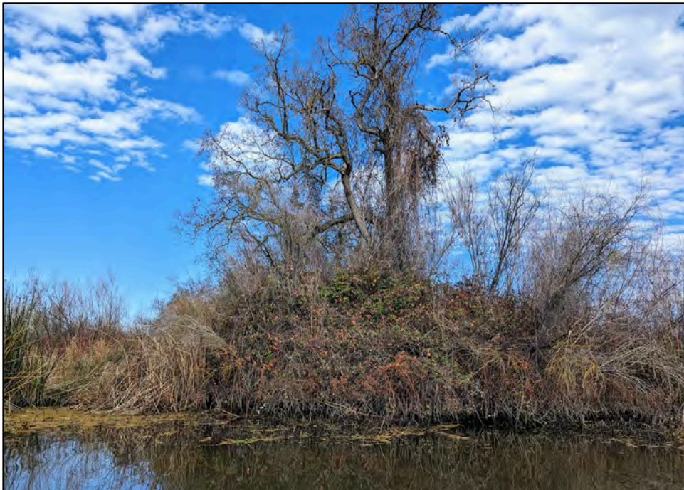
Photograph 5: The south end of the SLS 877 levee shows as an elevated mound heavily overgrown with brambles and topped with oaks and willows; facing north, February 8, 2024.
