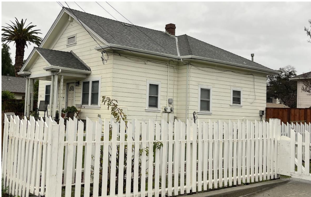
Figure 4. The building at 2086 Agnew Road, view of the north and west facades (Imagery date January 2023).
