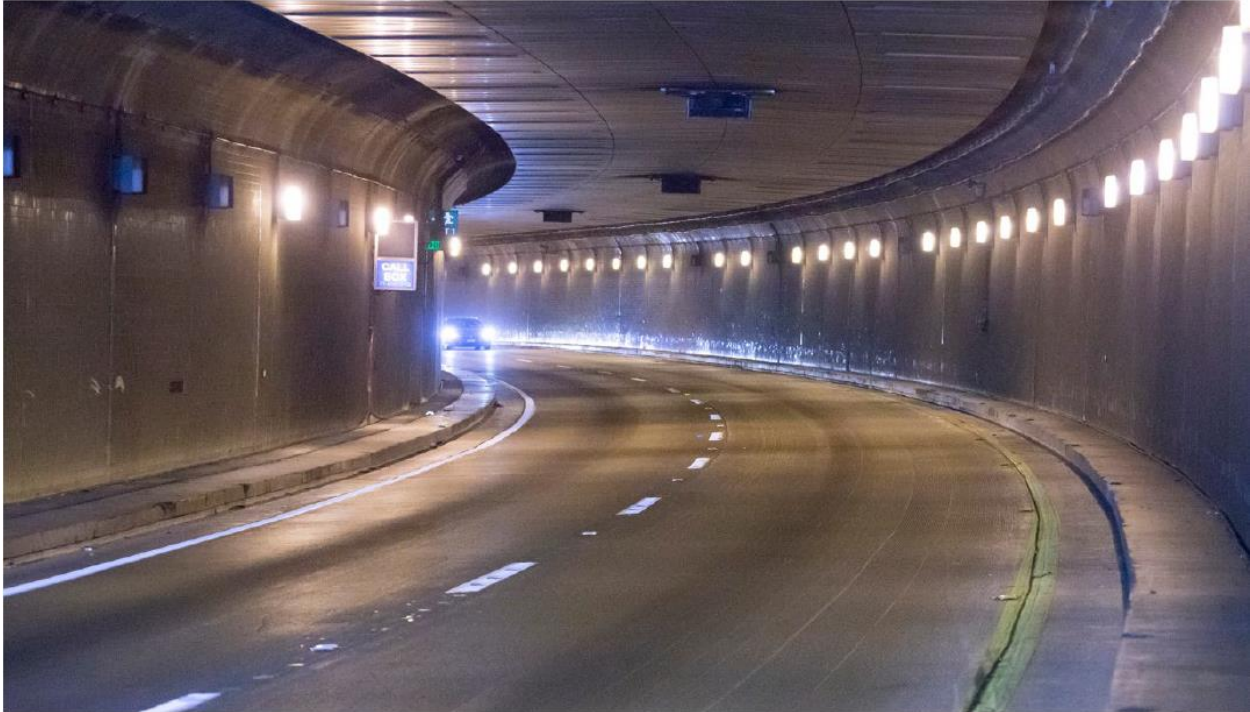
Figure 25. Existing view of Caldecott Tunnel Bore 3, eastbound.
