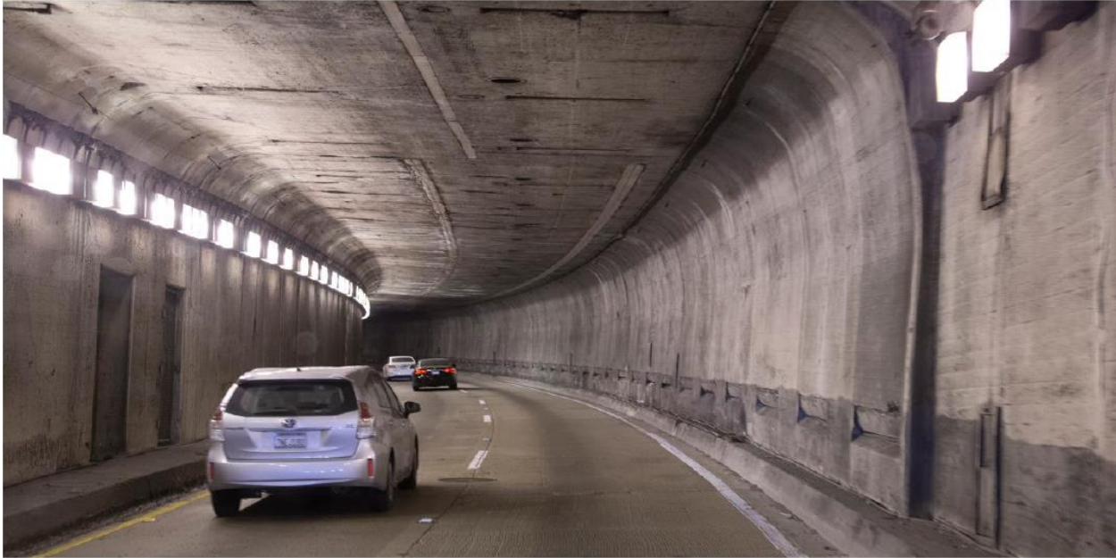
Figure 20. Existing view of Caldecott Tunnel Bore 1, eastbound.
