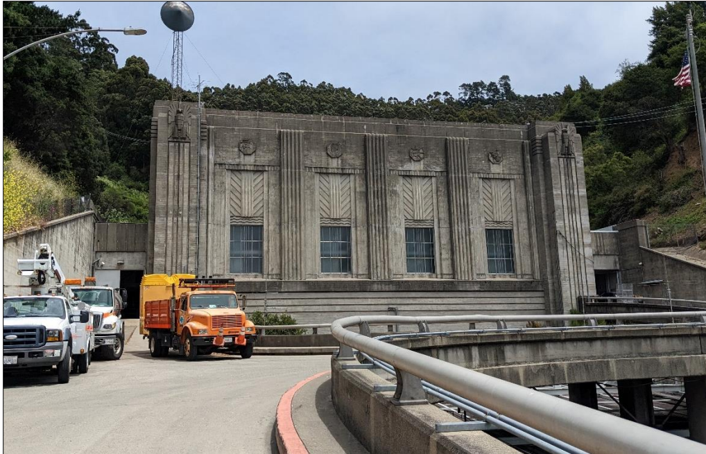
Figure 45. Caldecott Tunnel West Portal Building
