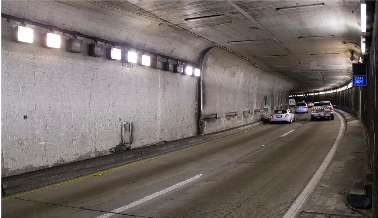
Figure 23. Existing view of Caldecott Tunnel Bore 2, eastbound.
