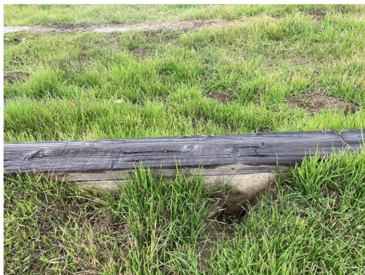
Photo 4 - West side of site; wooden plank on top of concrete foundation.
