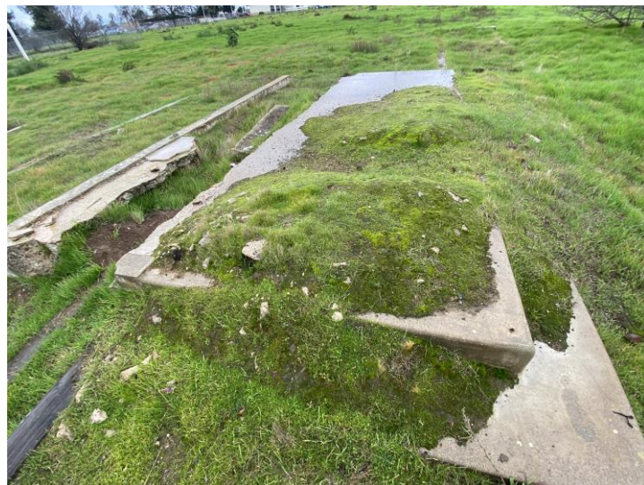
Photo 2 – Concrete slab/steps in west side of site.
