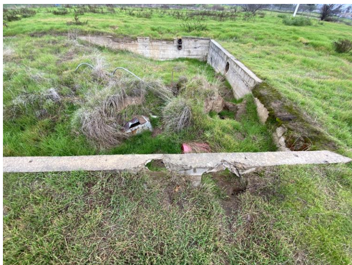
Photo 3 - Cellar in east side of site.
