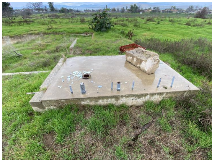
Photo 1 - Concrete slab in northeast corner of site.
