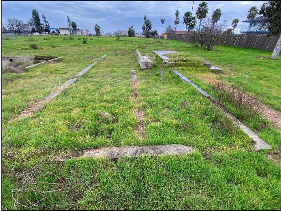
Figure 4-7 Foundations of demolished circa 1930-1940s rural residence, facing south.
