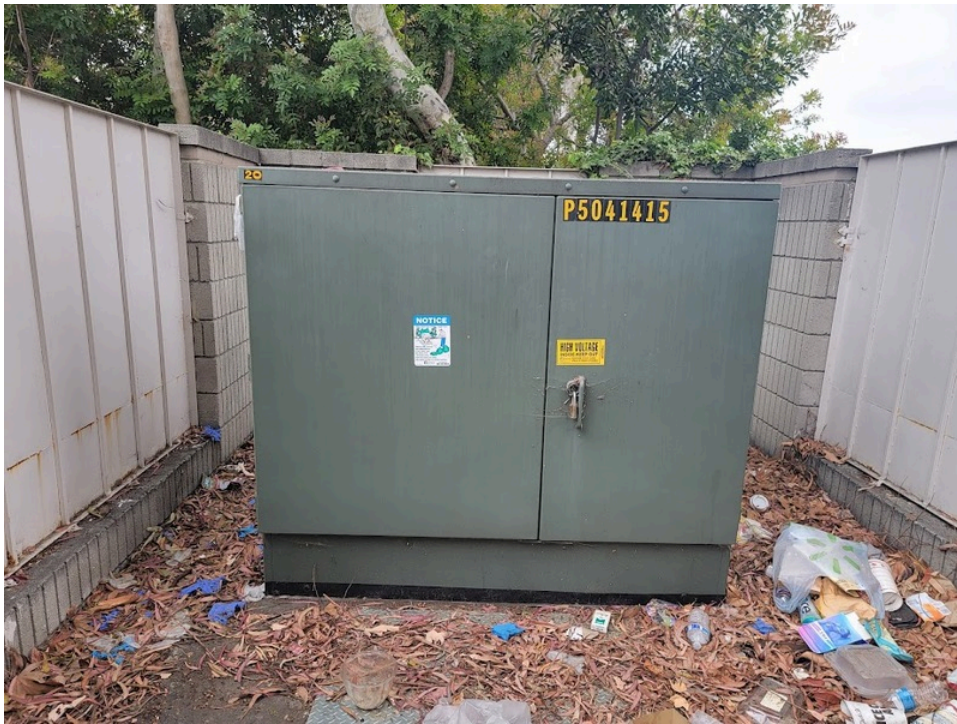
14. Pad-mounted transformer
