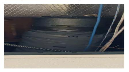
2. Fiberglass insulation w/wrap and tape.
