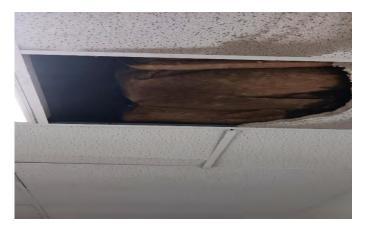
5. Fissured ceiling tile, fiberglass insulation.
