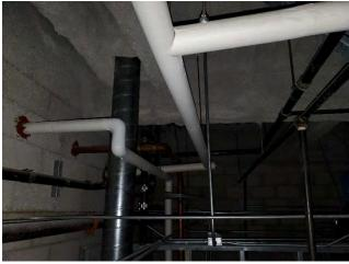
4. Fiberglass Pipe Insulation.
