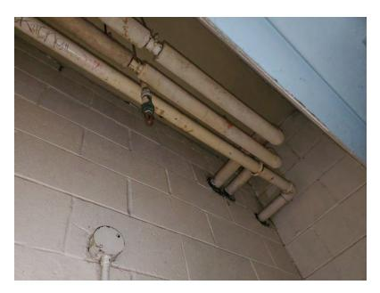
5. Example of fiberglass pipe run with ACM pipe elbows. (Hallway utility closet)
