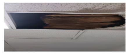
1. Fiberglass insulation and fissured ceiling tile.
