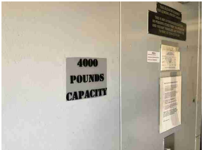
8) View of the capacity rating on the cab wall.
