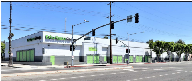
West and south elevations, view northeast (8/18/23)
