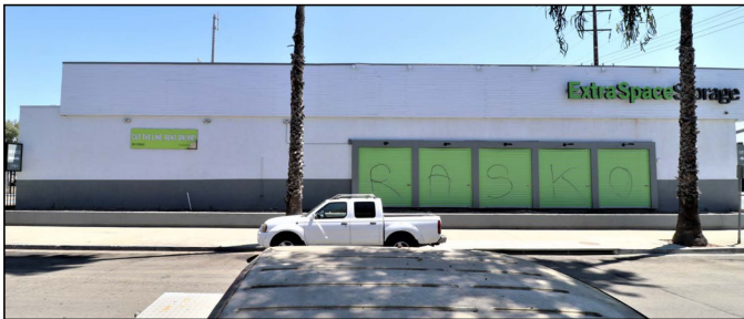
West elevation, view east (8/18/23)
