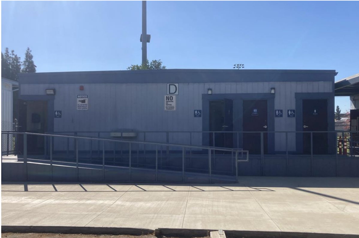
Figure 24 Restroom Building North Elevation, View South.
