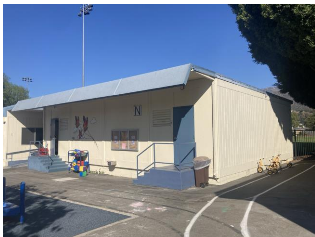
Photo 11: Example of Portable Classroom (Classroom N South and East Elevations), View Northwest
