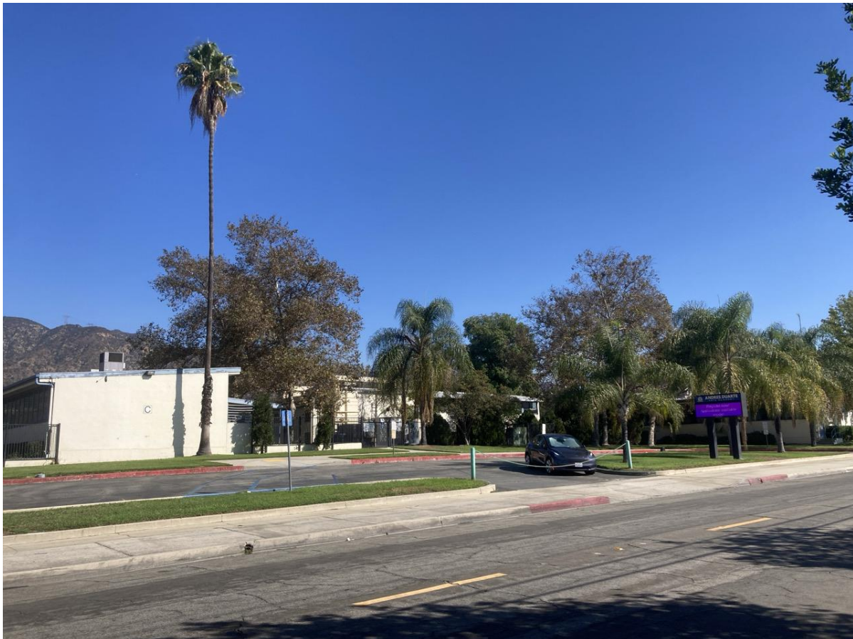
Figure 7 1433 Crestfield Drive, View Northeast
