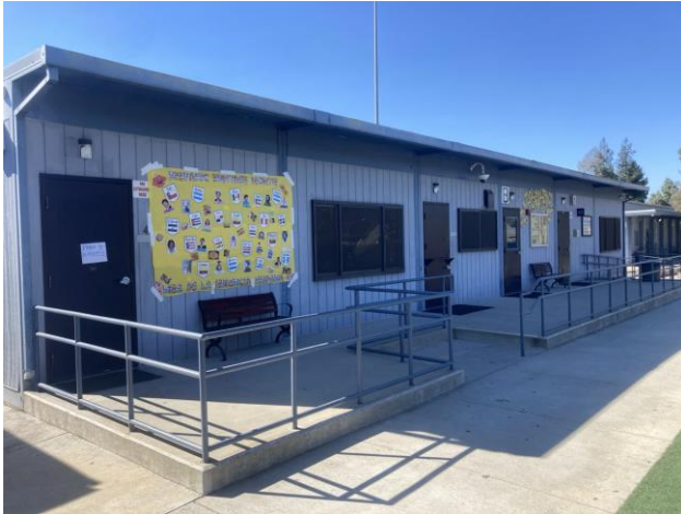
Photo 4: Administration Building North Elevation, View Southwest.
