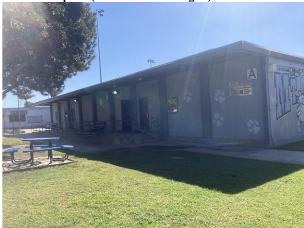
Photo 2: Classroom A North and West Elevations, View Southeast
