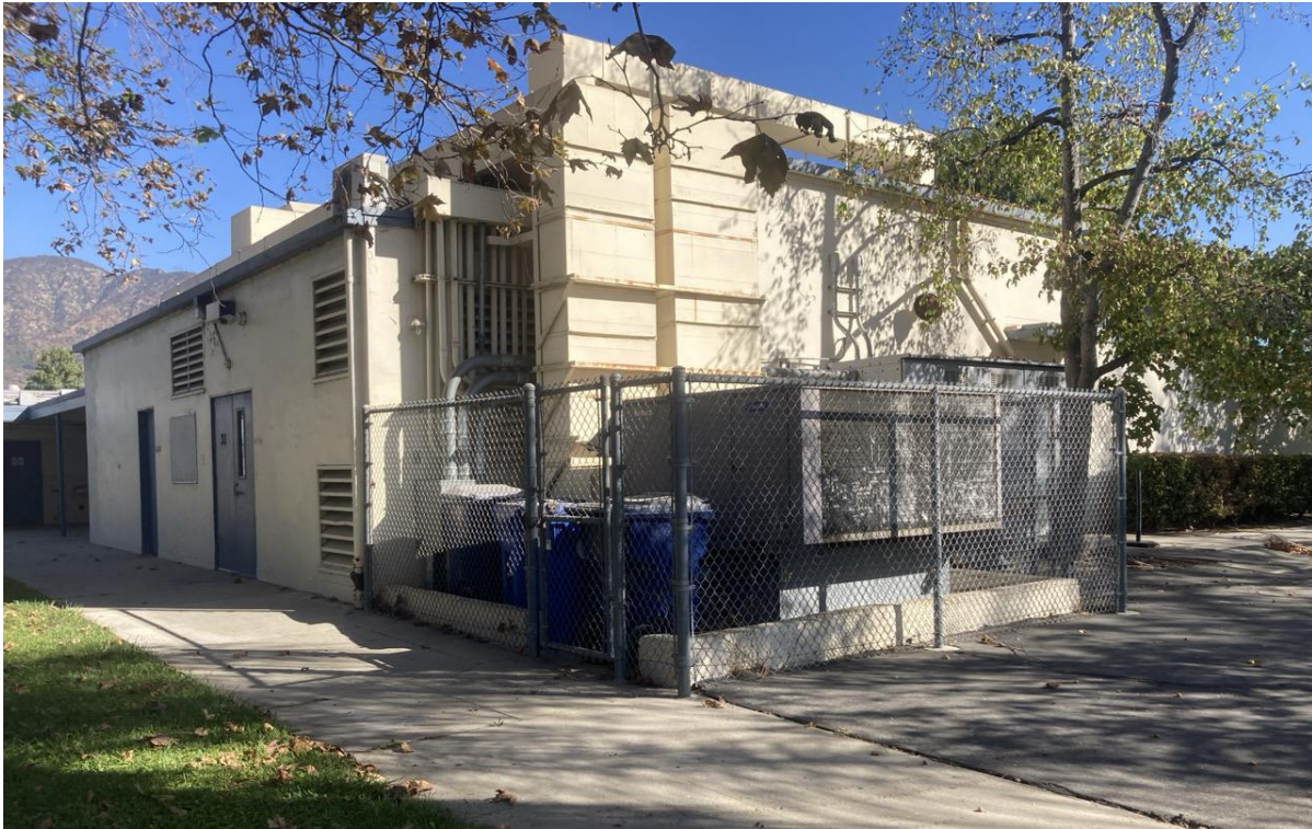
Figure 14 Multi-purpose Room South and West Elevations, View Northeast
