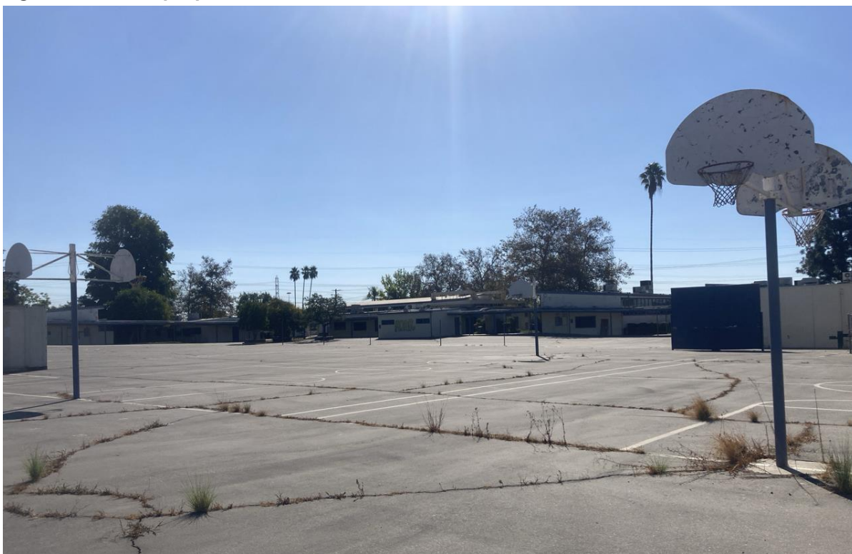
Figure 21 Paved play area and basketball court, View Southeast
