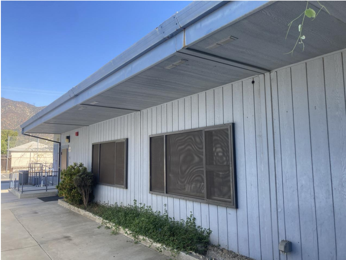
Figure 26 Classroom C West Elevation, View Northeast
