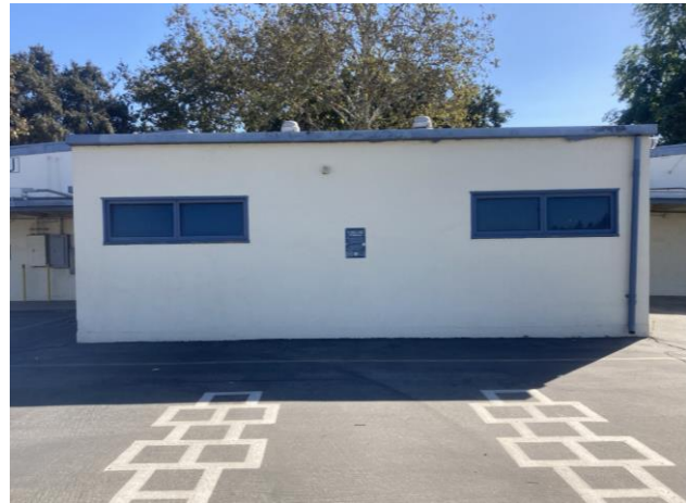
Photo 7: Representative Photograph – Rear Elevation of Restroom Buildings, View East.
