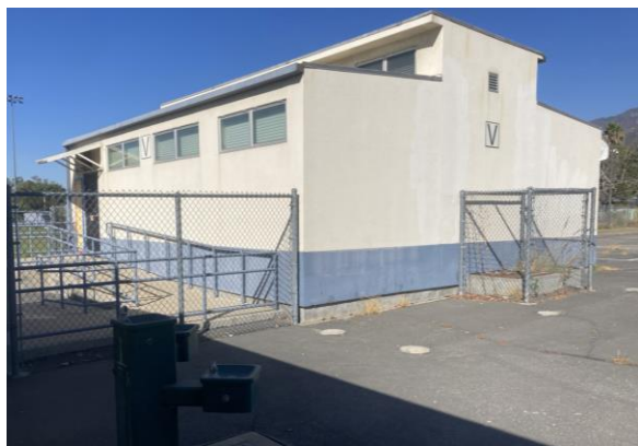
Photo 13: Offices South and East Elevations, View Northwest
