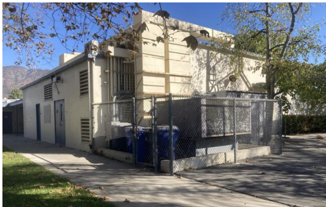
Photo 8: Multi-purpose Room South and West Elevations, View Northeast.
