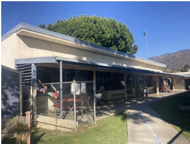
Photo 2: Representative Photograph – Primary Elevation of Classroom A, View Northwest.
