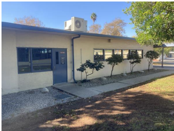
Photo 9: Administration Building North Elevation, View Southwest.
