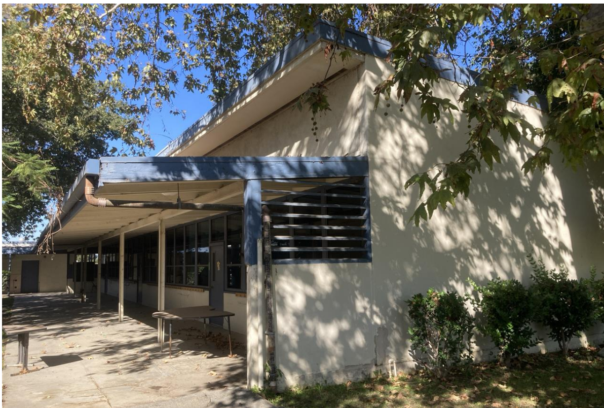
Figure 10 Representative Photograph – Primary and East Elevations of Classroom J, View West
