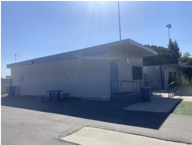
Photo 6: Classroom E North and West Elevations, View Southeast.
