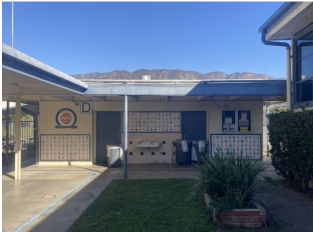
Photo 6: Representative Photograph – Primary Elevation of Restroom Buildings, View North.
