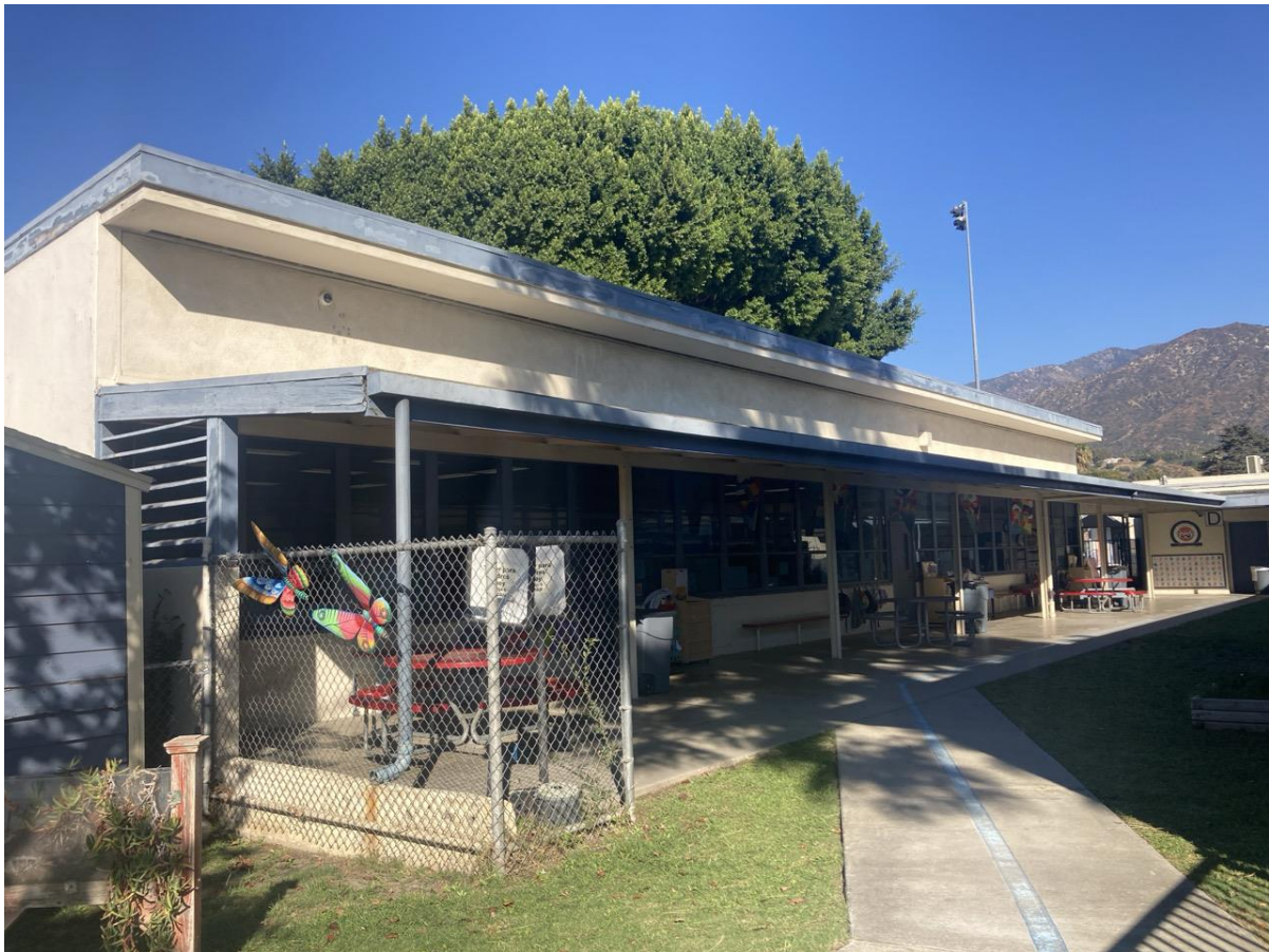
Figure 8 Representative Photograph – Primary Elevation of Classroom A, View Northwest
