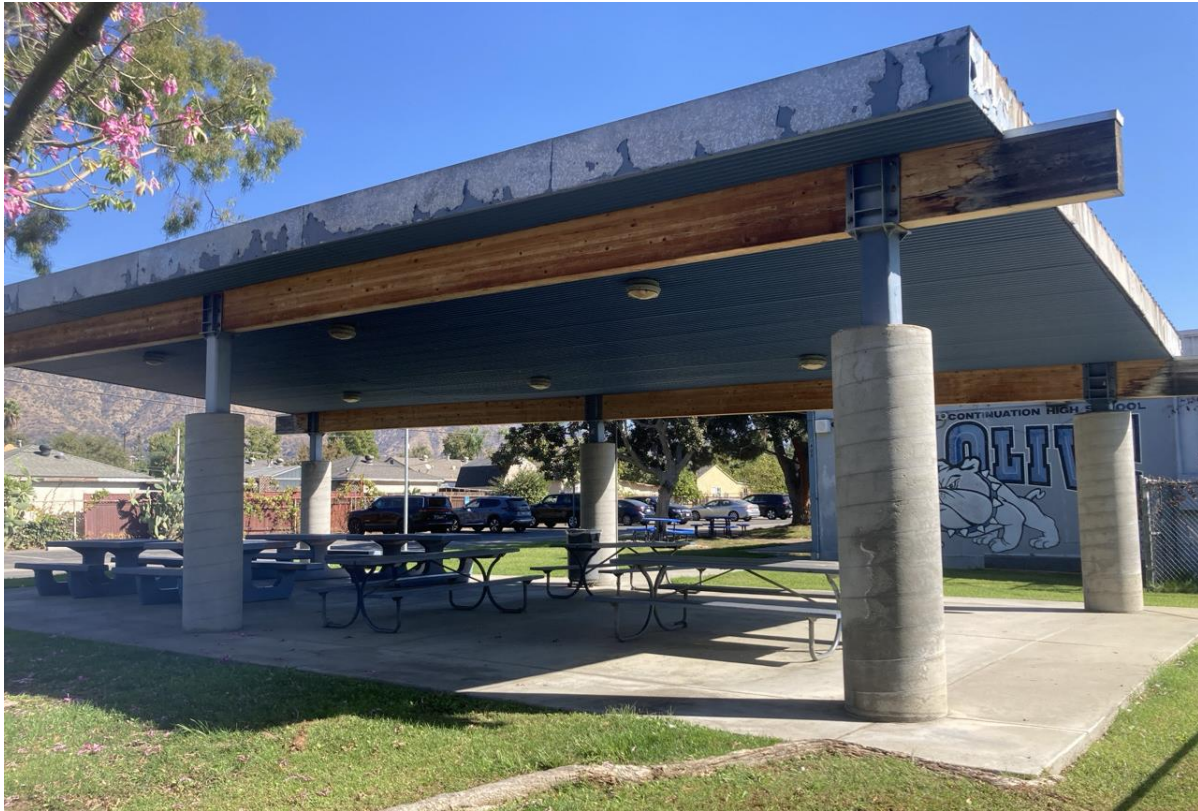
Figure 28 Open Lunch Structure, View Northeast
