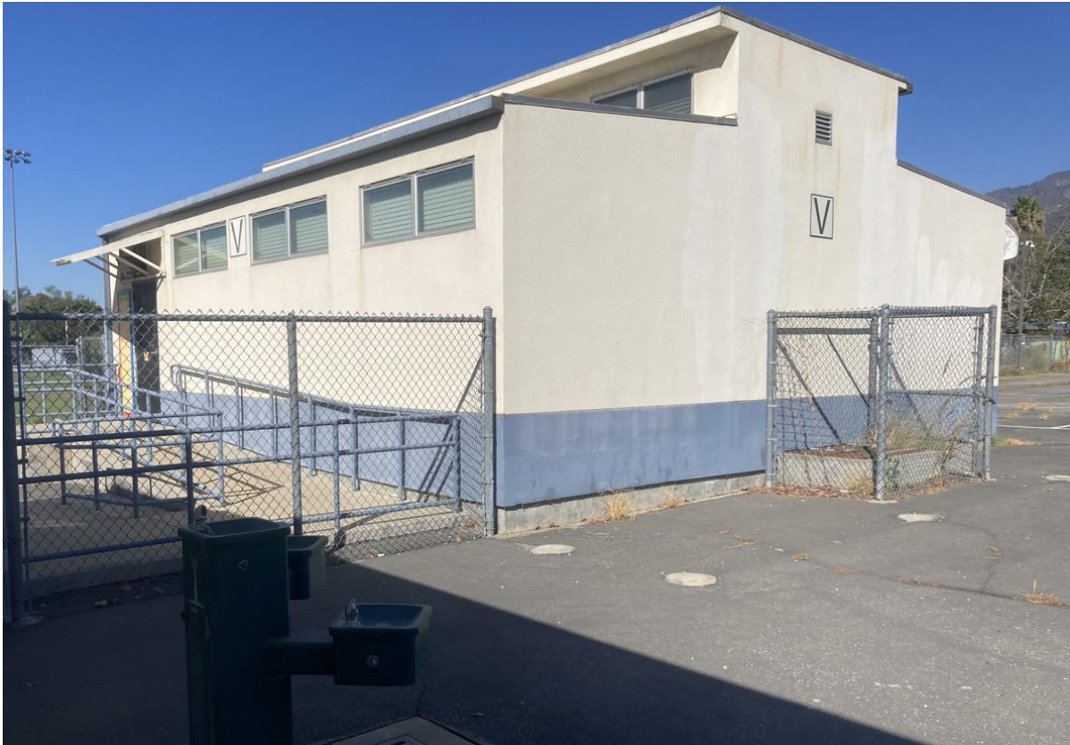
Figure 19 Offices South and East Elevations, View Northwest
