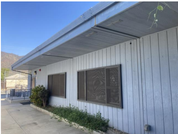
Photo 5: Classroom C West Elevation, View Northeast.
