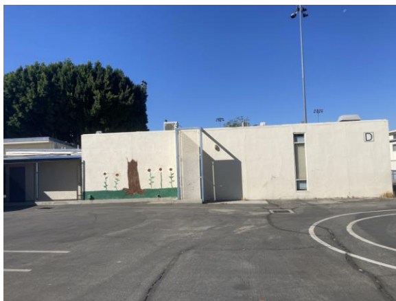
Photo 10: Locker Rooms East Elevation, View West.
