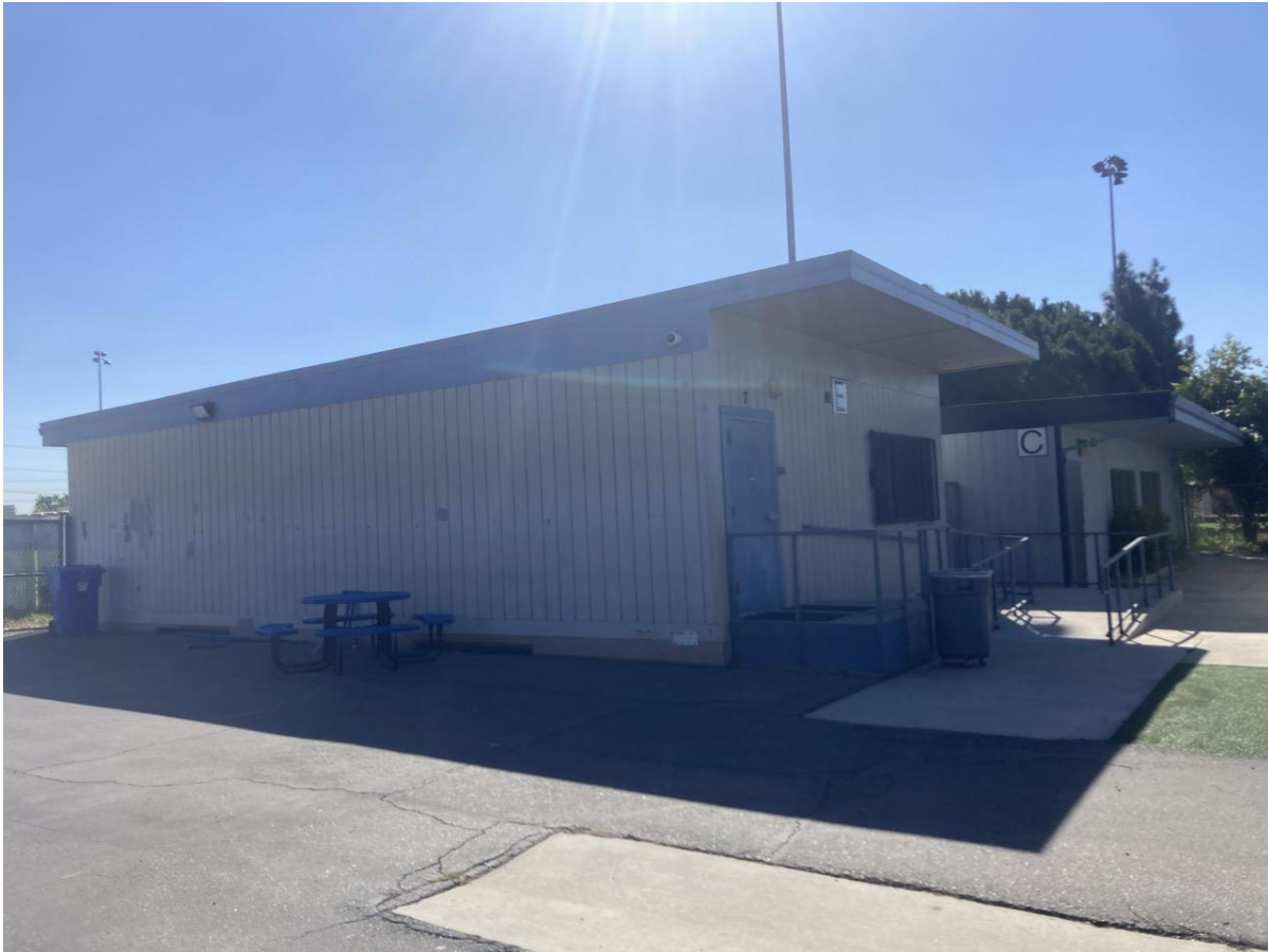
Figure 27 Classroom E North and West Elevations, View Southeast.
