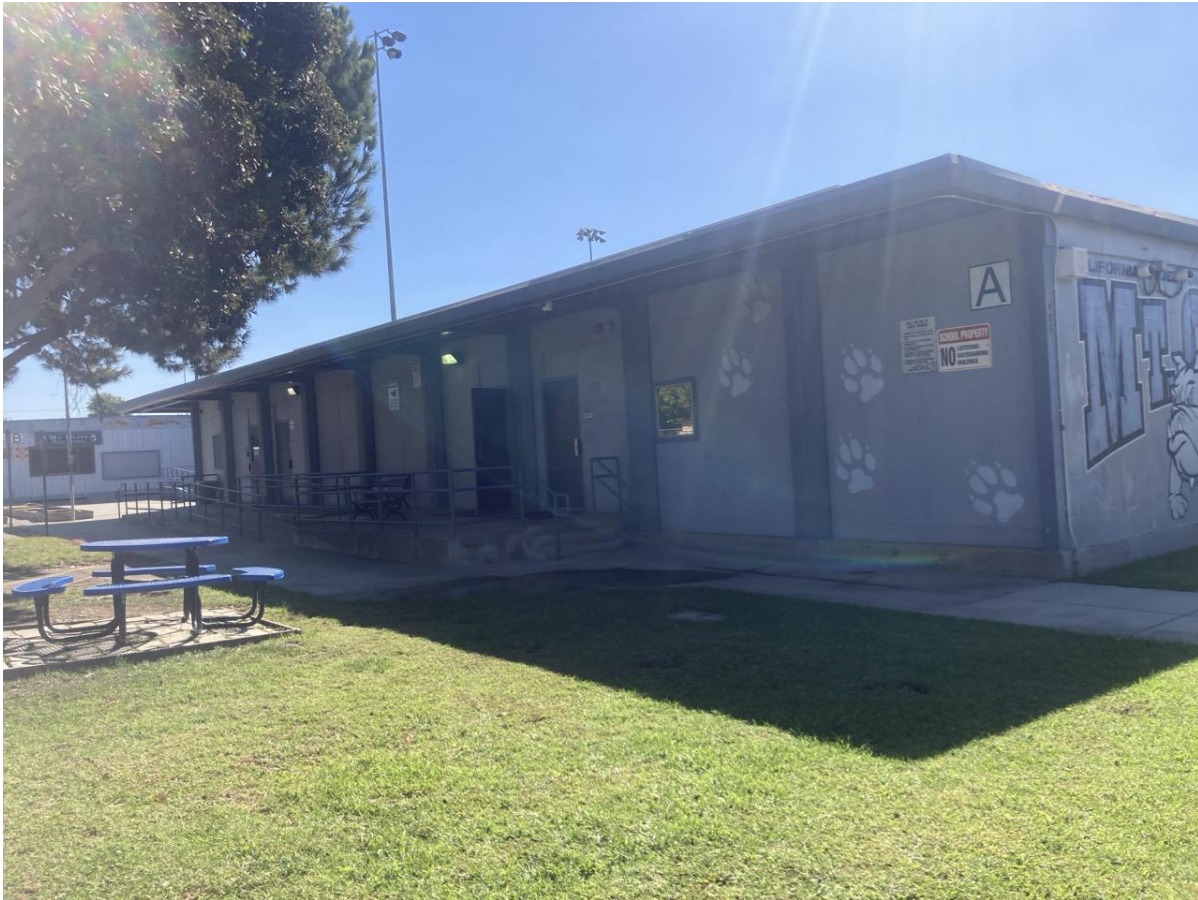
Figure 23 Classroom A North and West Elevations, View Southeast
