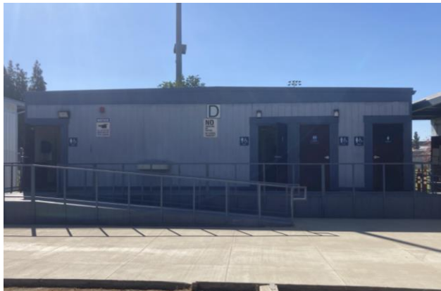
Photo 3: Restroom Building North Elevation, View South.
