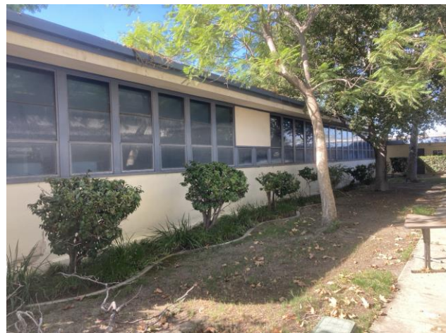
Photo 5: Representative Photograph – Rear Elevation of Classroom I, View Southwest.
