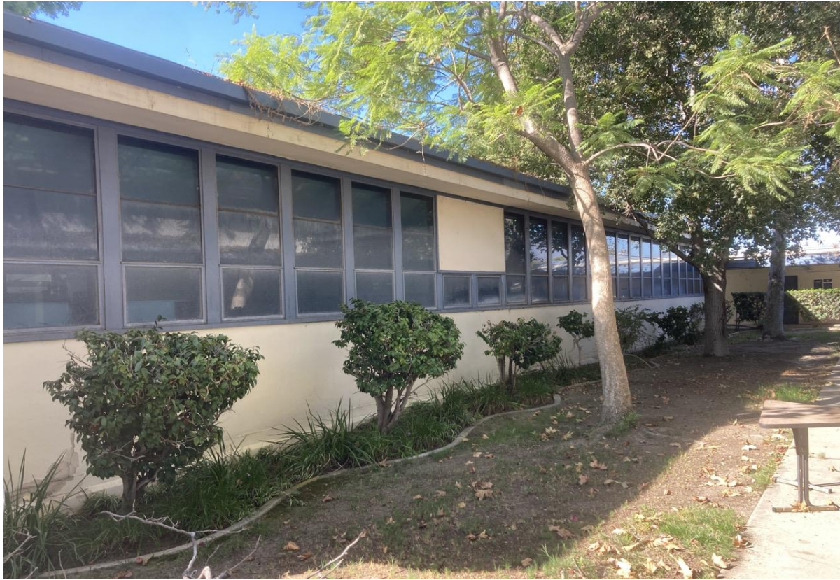
Figure 11 Representative Photograph – Rear Elevation of Classroom I, View Southwest
