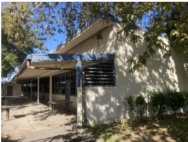
Photo 4: Representative Photograph – Primary and East Elevations of Classroom J, View West.
