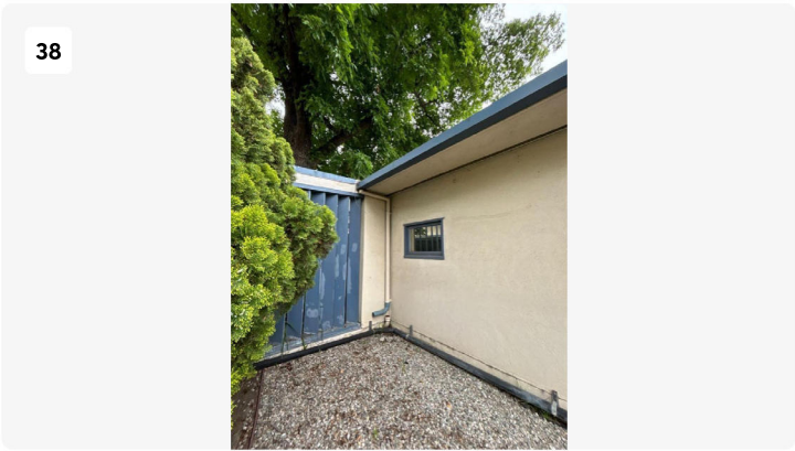
Building H positive gutter, downspout
