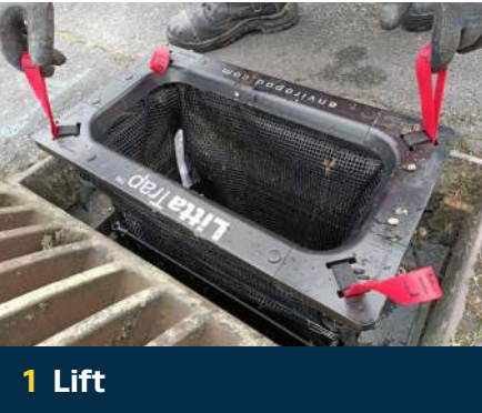
Lift the LittaTrap™ FC out of the catch basin using the LIFT handles
