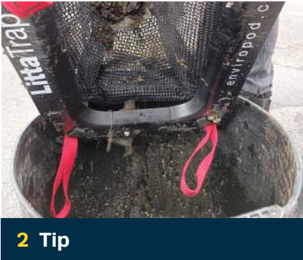
Tip the contents out of LittaTrap™ FC into suitable receptacle for contents
