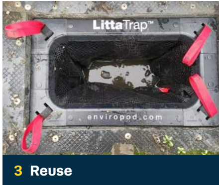
Reuse the LittaTrap™ FC by placing securely back into the surrounding frame and seal, and close grate.
