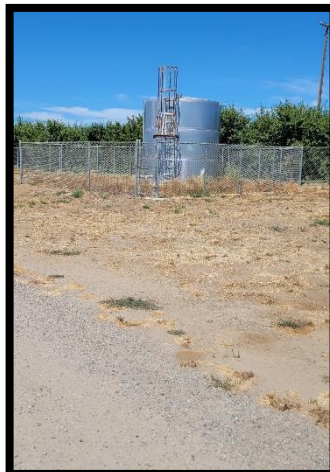
Photo 5: Looking Northwest at the static tank located along the eastern property line of Stanislaus Elementary School.
