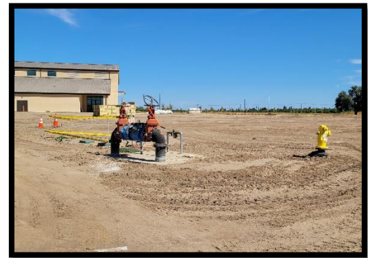
Photo 6: Looking East at on-going construction within the parcel on the east side of Tully Road.
