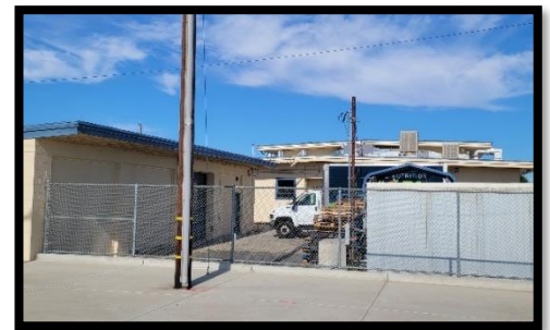
Photo 12: Looking Northeast towards the buildings directly north of Stanislaus Elementary School drop-off line and parking lot.
