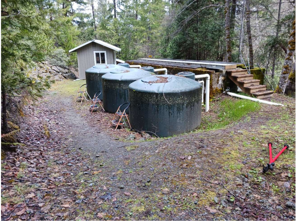
Figure 7: Existing water treatment facility
