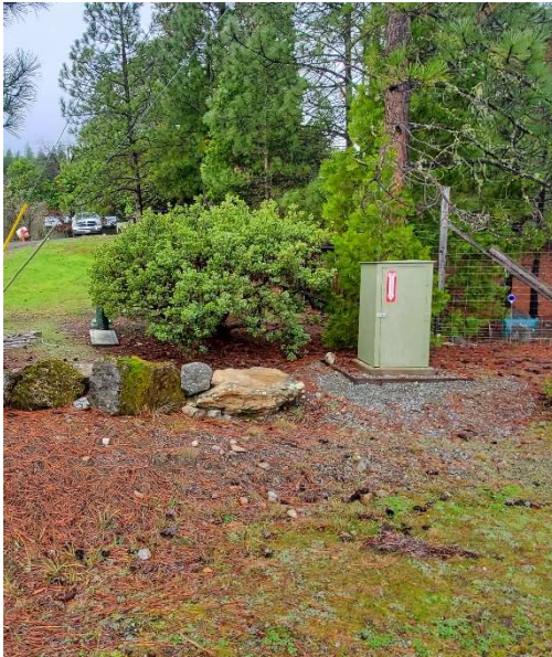
Figure 5: Typical existing fire hydrant and water meter scheduled to be replaced.
