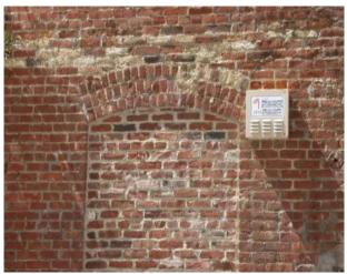
Figure 16. Close-up view of filled-in brick doorway.
