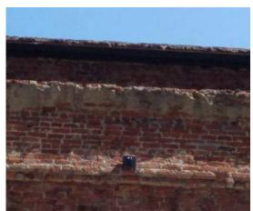
Figure 36. Close-up of patched bricks at belt course where cornice was damaged.
