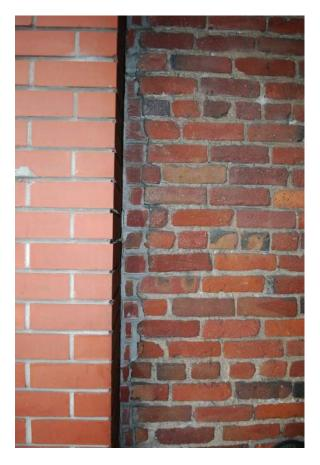
A comparison between the new brick of 1967 (far left) and the old brick of 1906-1907 (at right). This view is in one of the recessed entrances of the main facade.
