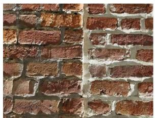
Figure 37. Close-up of bricks showing areas that were recently sandblasted (right) and not (left).
