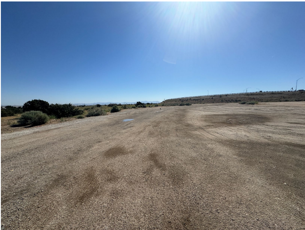
Figure 5: Overview of Grading in the Southwestern Portion of the Project Area
