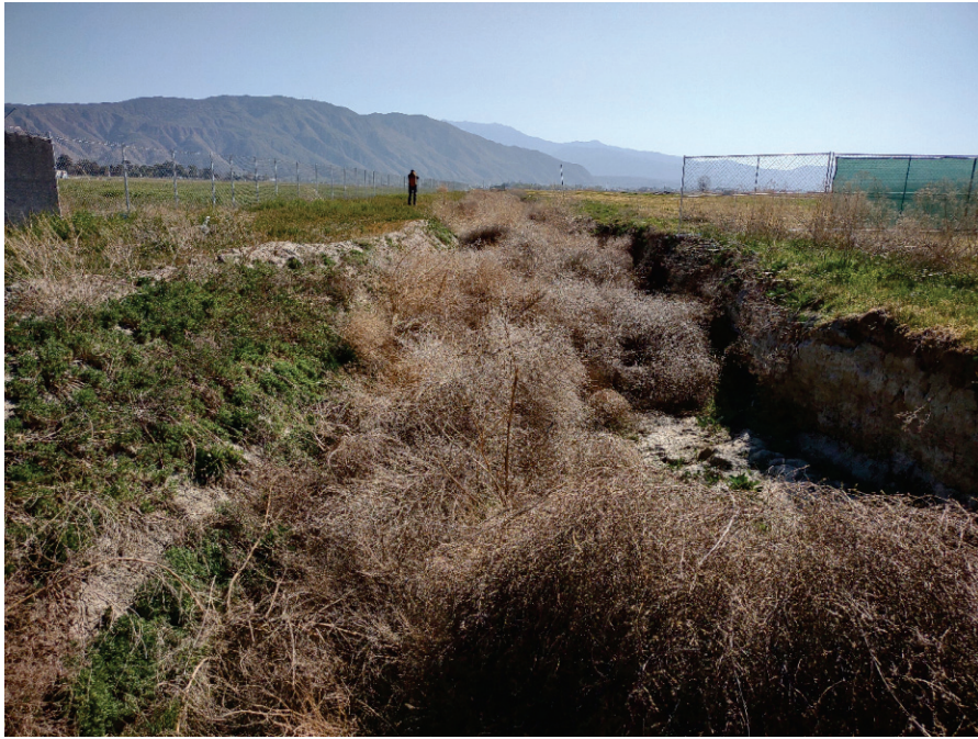
Photo 3: View of Feature 1 condition, vegetation present within its bed and banks and adjacent chain link fences. Facing southeast. Taken on March 16, 2022.
