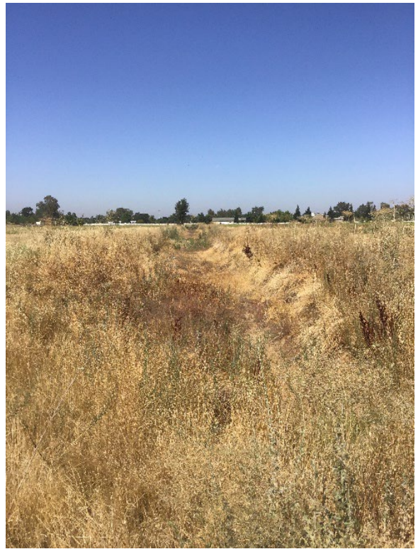
Drainage canal in center of Project site. Take on the dirt road crossing the canal, facing west.
