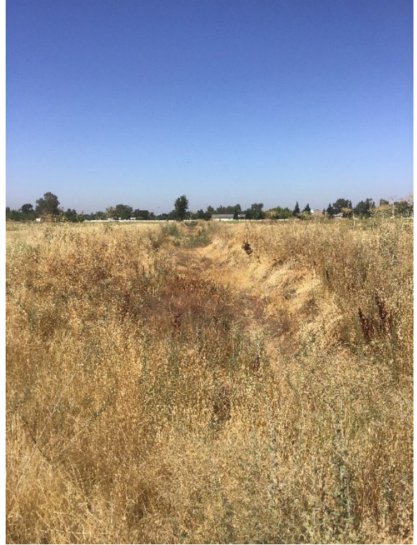
Photo Point 2. Drainage canal in center of Project site. Take on the dirt road crossing the canal, facing west.
