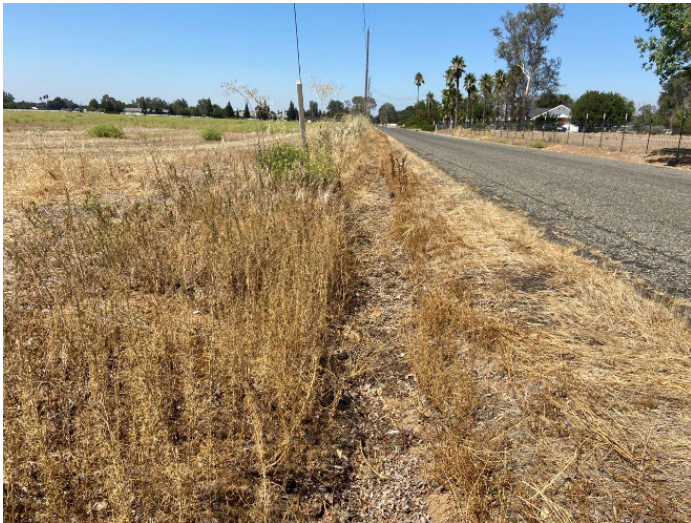
Photo Point 7. Roadside ditch along northern boundary of Project site. Facing west.
