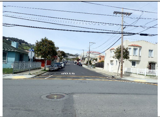
Typical view of developed area in the residential area between the Cow Palace property and the PG&E Martin Substation
