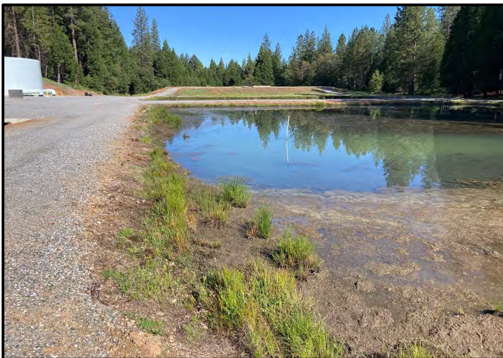
East backwash pond, looking northwest; 05/15/24.
