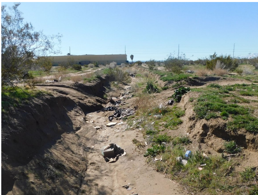
Photograph 2: From the terminus of on-site portions of Drainage A looking south (upstream).
