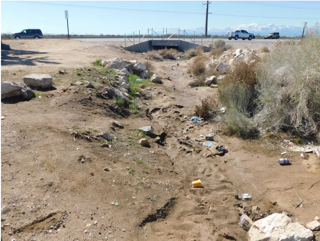
Photograph 3: Upstream (south) of the off-site street improvement area, Drainage A originates at a box culvert beneath Palmdale Road.
