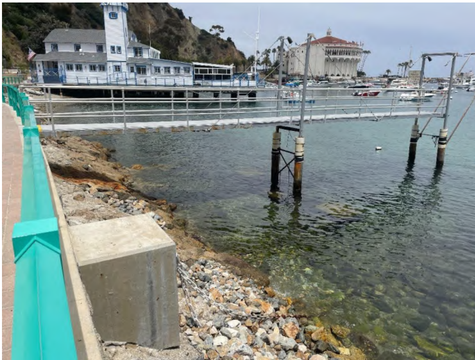
Photograph 3. South side of dock pilings; view to north.
