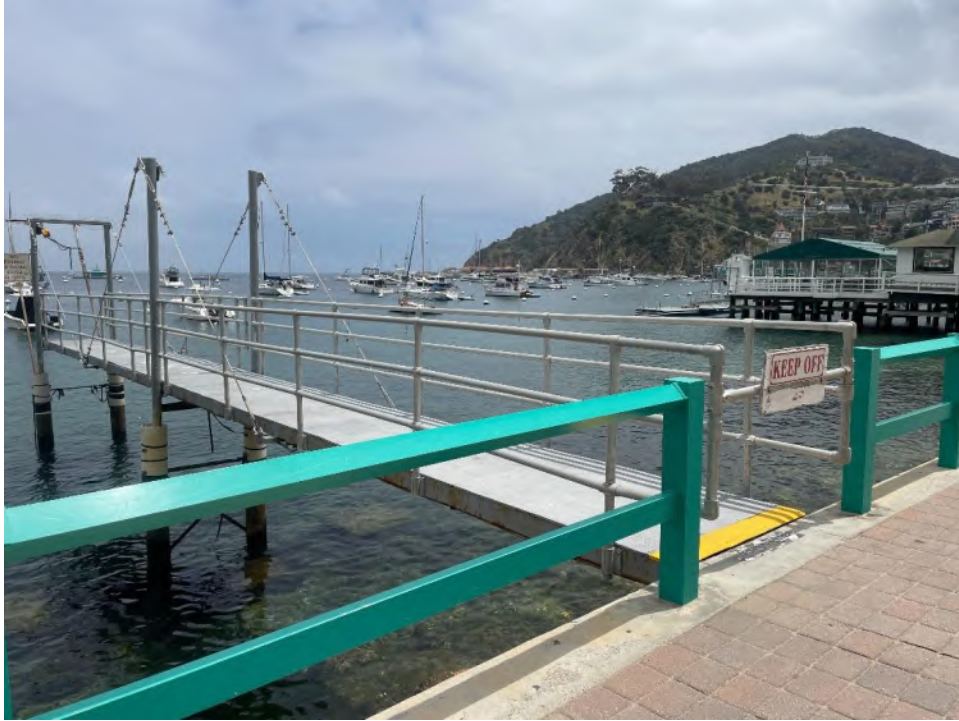
Photograph 6. Attachment of dock to seawall; view to east.
