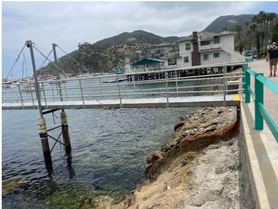
Photograph 5. North side of dock attachment to seawall; view to south.
