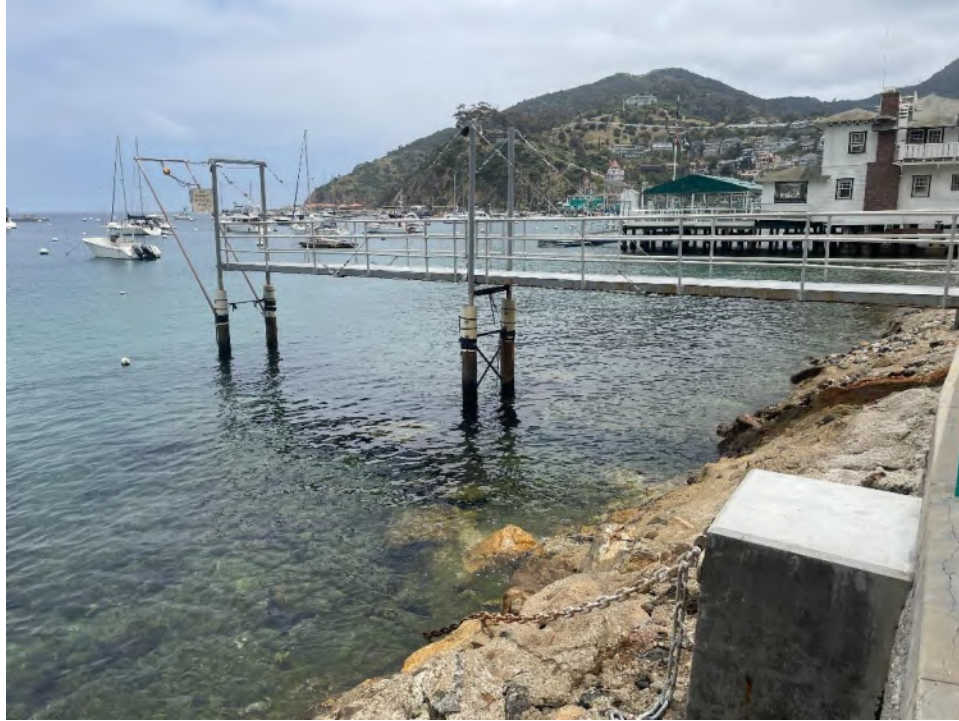
Photograph 4. North side of dock pilings; view to southeast.
