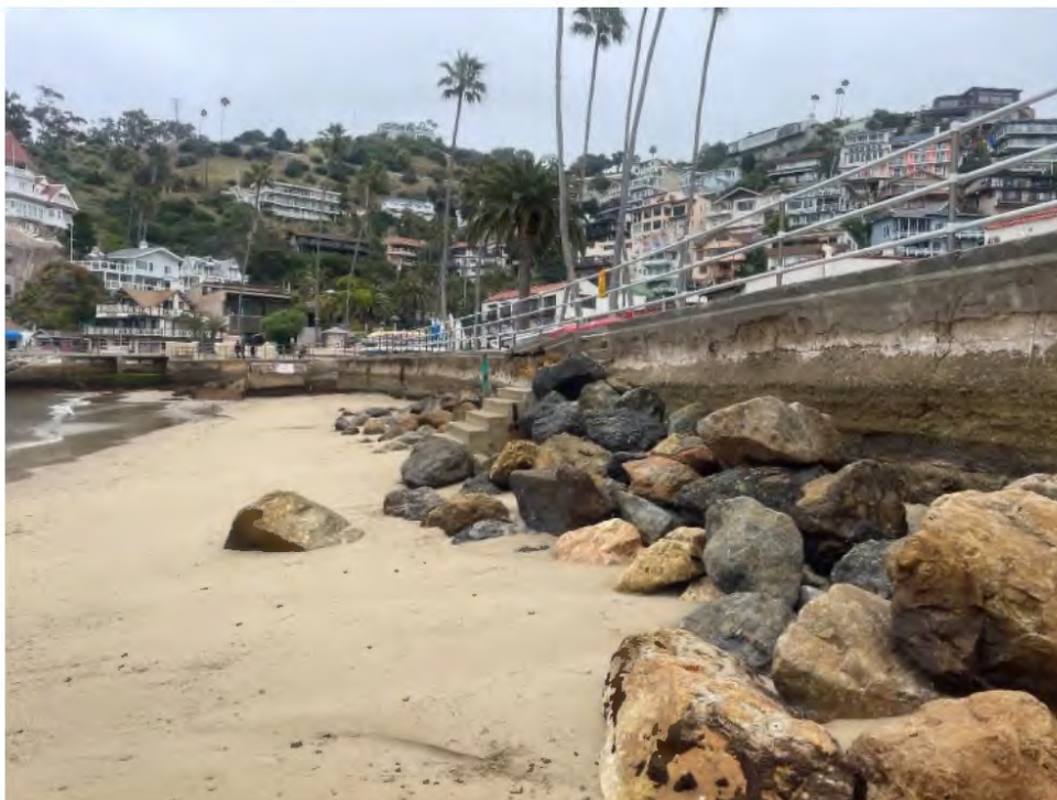
Photograph 2. Overview of South Beach Seawall, view to southeast
