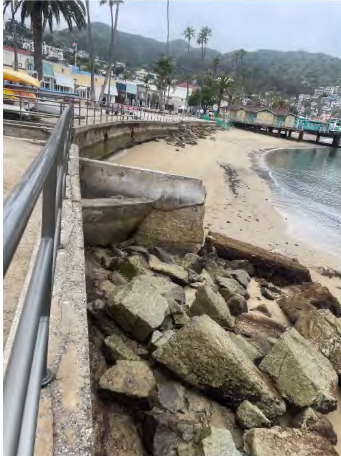
Photograph 3. Groin Wall, view to west
