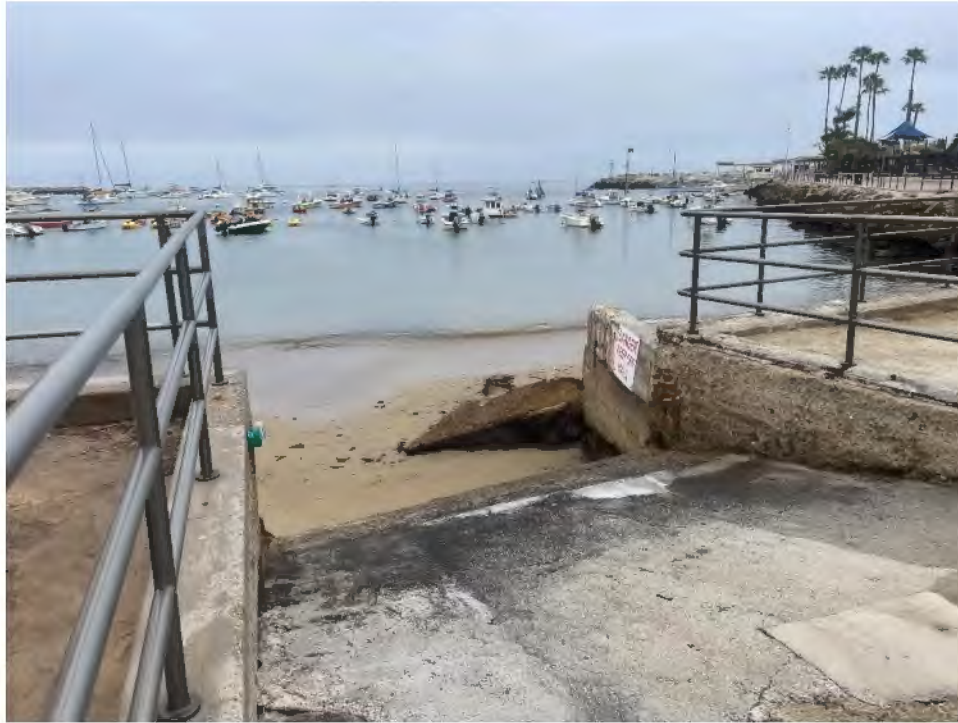
Photograph 2. Boat ramp, view to northeast
