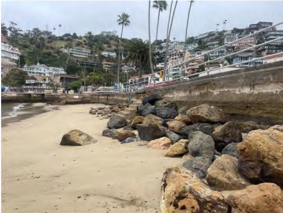
Photograph 1. Overview of South Beach Seawall, view to southeast
