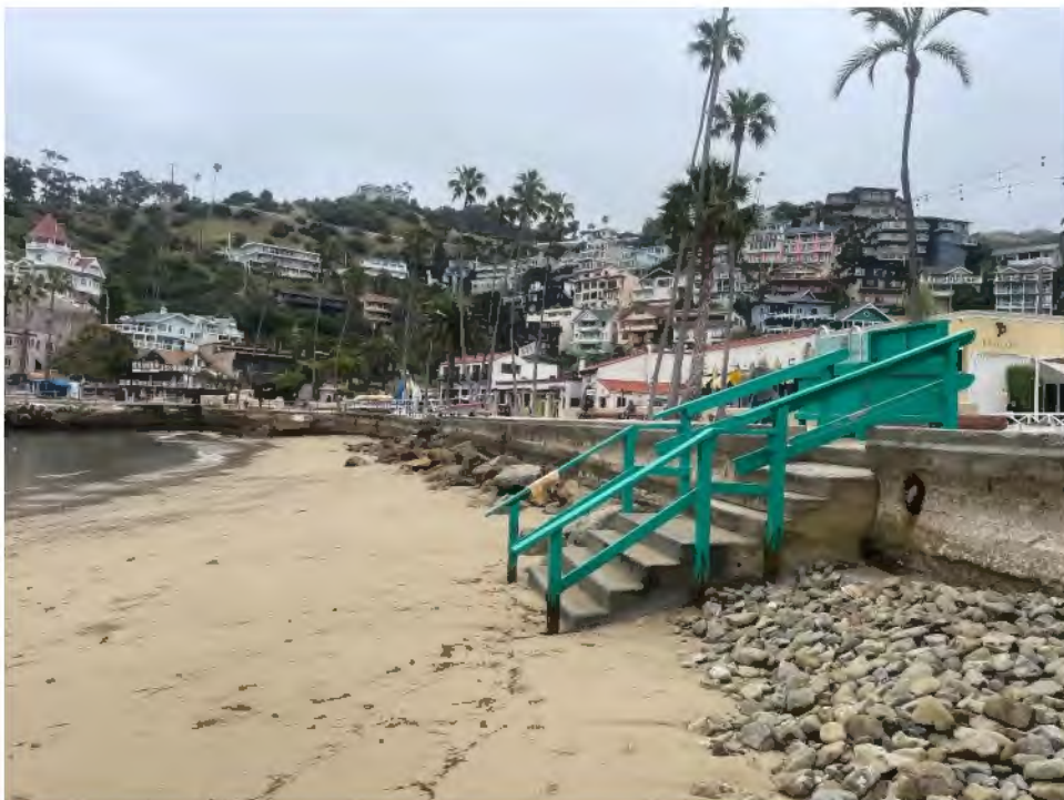
Photograph 5. Beach access staircase and Seawall, view to southeast
