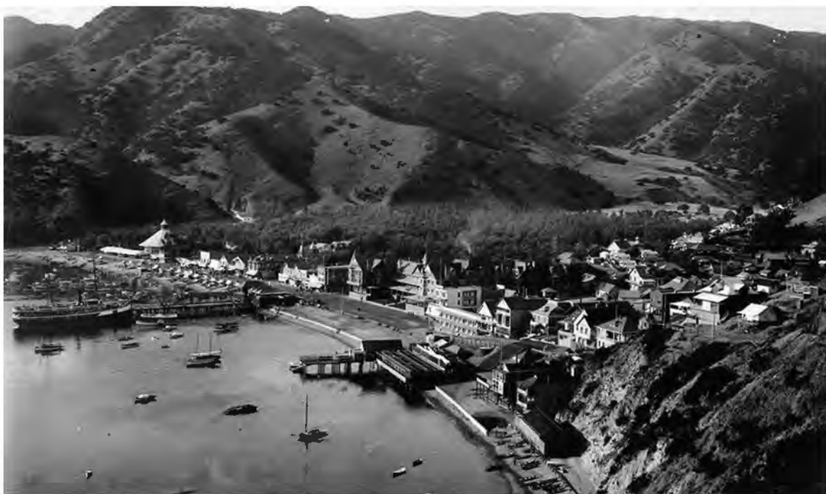
Exhibit 1. Circa 1906 photograph of the Avalon Bay coastline showing denser development and seawalls on the northern shoreline (foreground) and sparse development on the southern shoreline (Austin's Catalina Historical Archives (ACHA) 2024).
