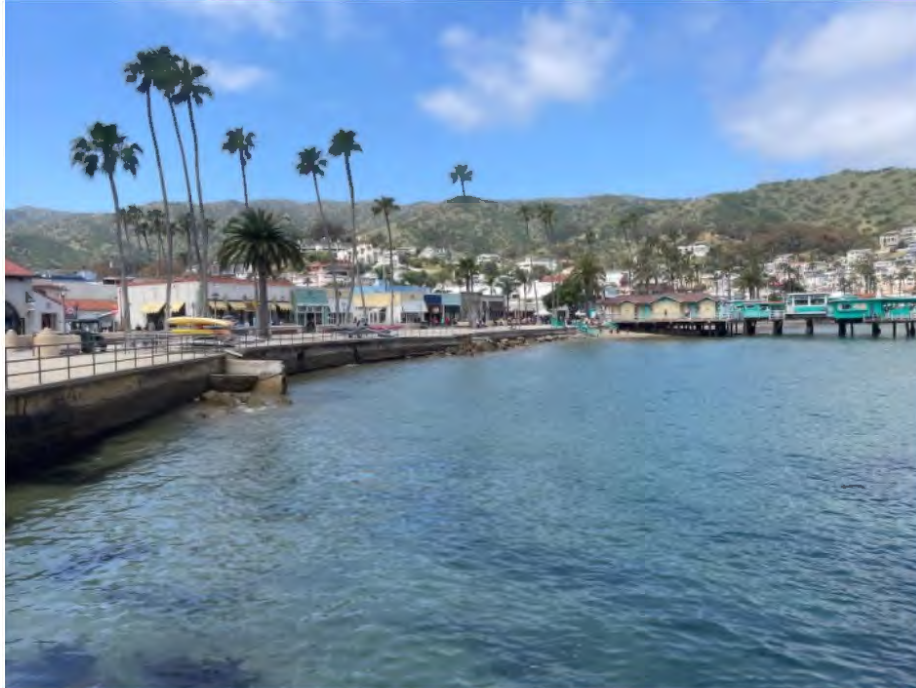
Photograph 1. Overview of South Beach Seawall, view to west
