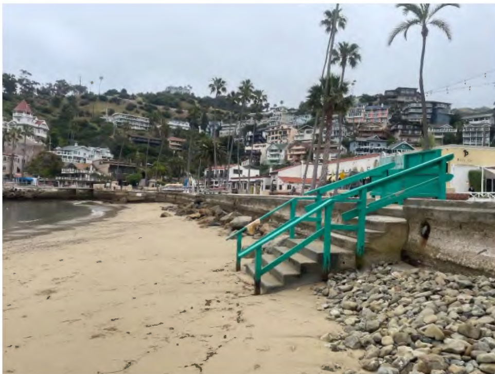
Photograph 6. Beach access staircase and Seawall, view to southeast
