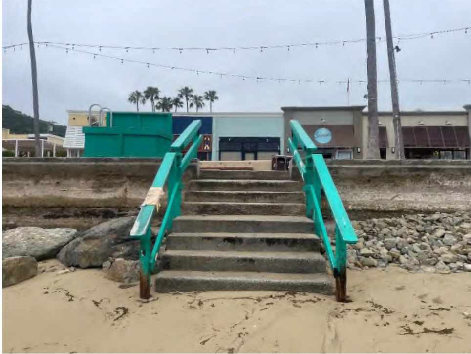
Photograph 7. Northernmost staircase, view to southwest
