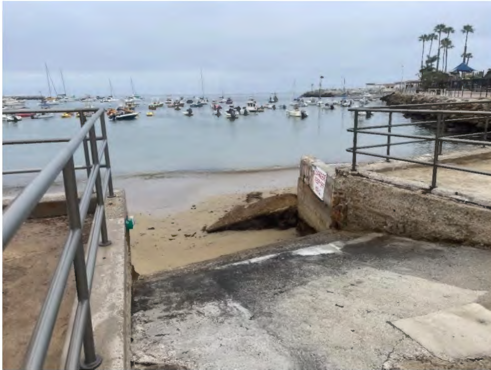
Photograph 3. Boat ramp, view to northeast
