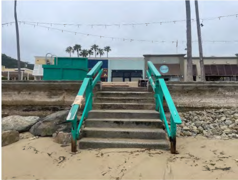
Photograph 6. Northernmost staircase, view to southwest
