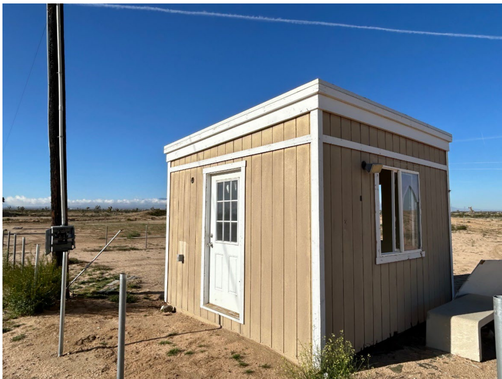
Overview of building on west parcel. View to west.
