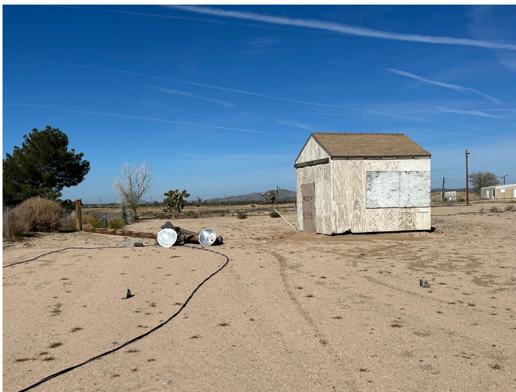
Overview of building on west parcel. View to west.
