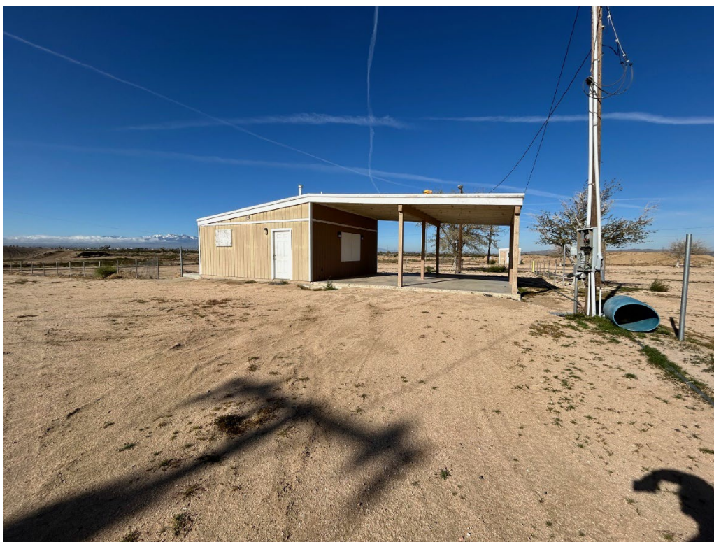
Overview of building on west parcel. View to southwest.
