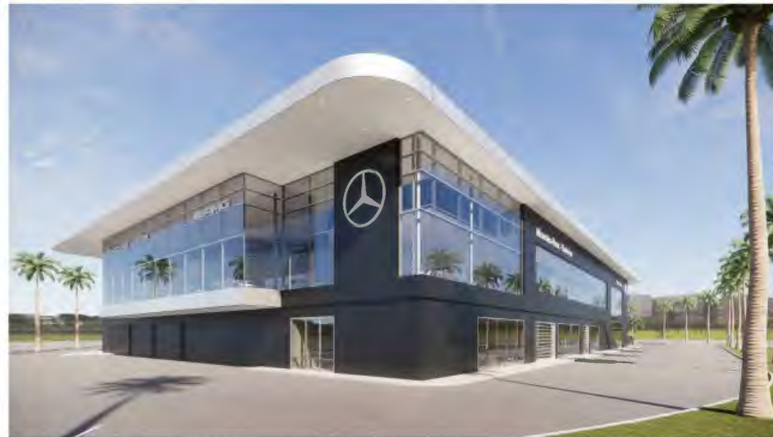
NORTH - FREEWAY VIEW - DAY
