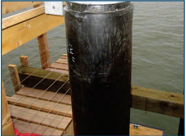
PROPOSED PILE STEEL W/ BLACK POLY SLEEVE 2
