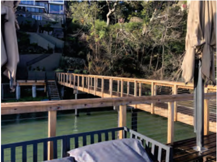
EXISTING GUARD RAIL CEDAR POSTS AND CAP W/ STAINLESS CABLES
