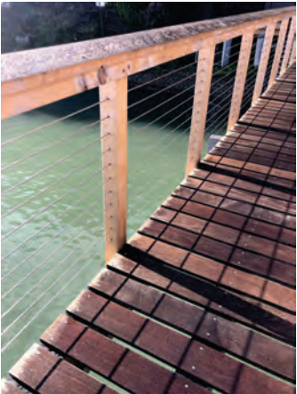
EXISTING GUARD RAIL CEDAR POSTS AND CAP W/ STAINLESS CABLES
