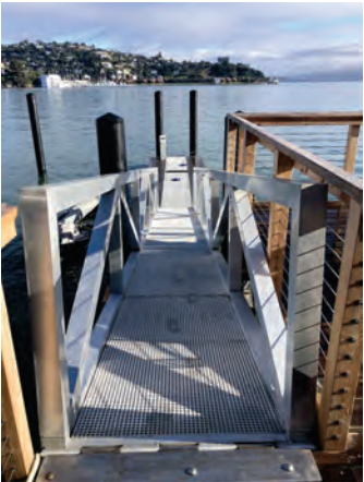
EXISTING GANGWAY ALUMINUM W/ TRHU FLOW DECK
