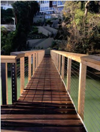
EXISTING GUARD RAIL CEDAR POSTS AND CAP W/ STAINLESS CABLES
