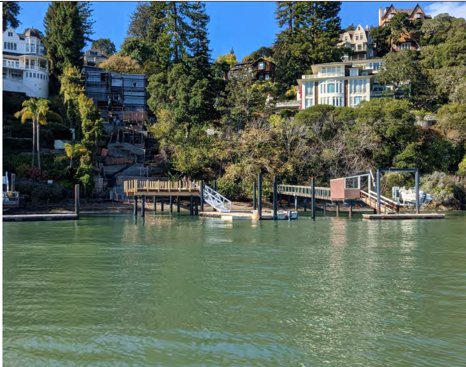
Photograph 4. Photo of the constructed pier and floating dock, October 29, 2021
