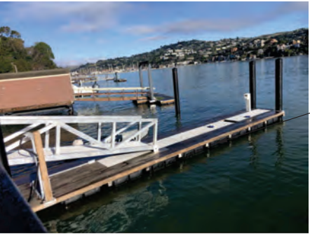
EXISTING GANGWAY ALUMINUM W/ TRHU FLOW DECK
