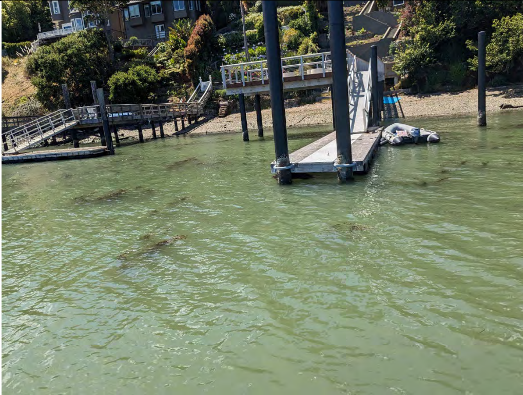
Photograph 5. Photo of the constructed pier and floating dock, July 24, 2023. Note eelgrass bed present and visible at the surface. More eelgrass is subsurface and is not visible.
