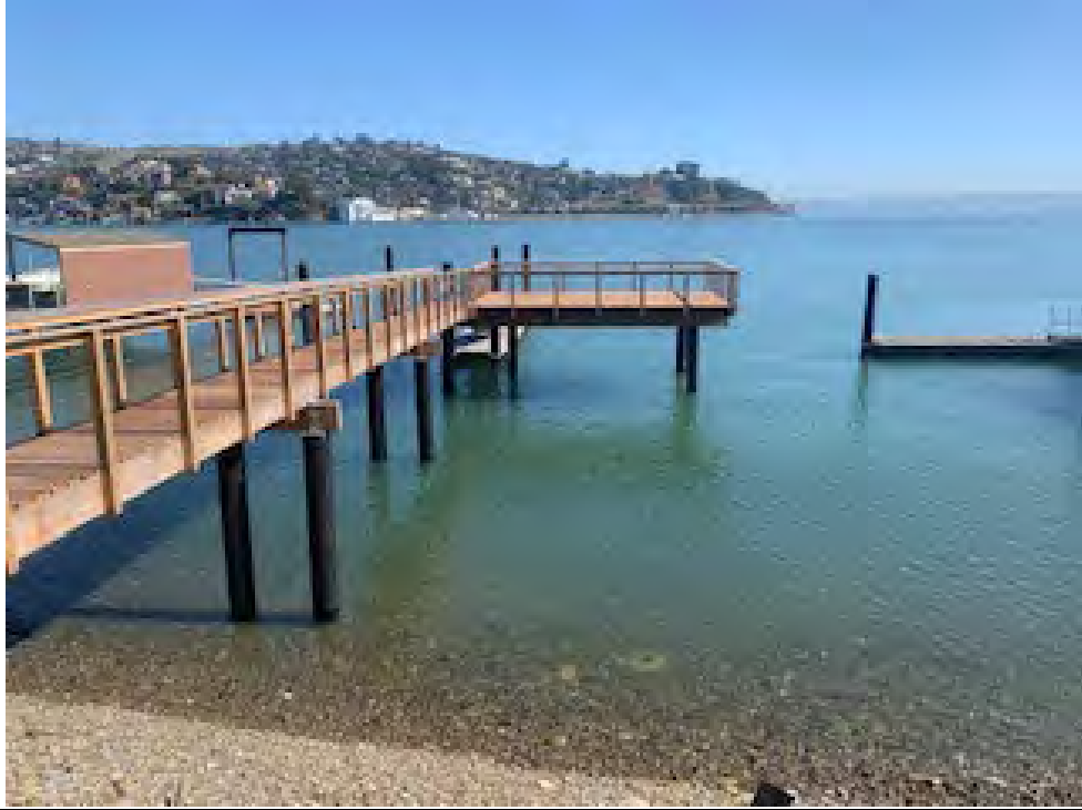
Photograph 3. Photo of the constructed pier and floating dock, October 29, 2021
