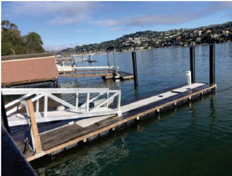
EXISTING GANGWAY ALUMINUM W/ TRHU FLOW DECK
