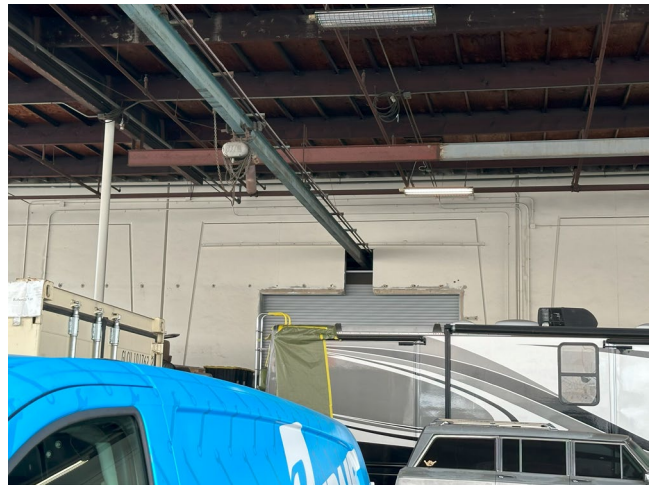
Westerly Bldg alteration detail, view E
