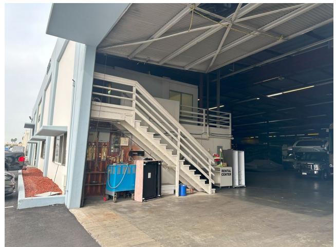
Easterly Bldg interior office, view NW
