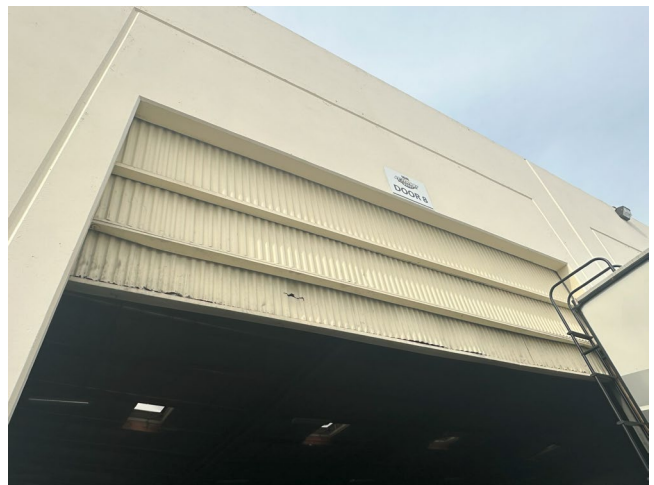
Westerly Bldg original telescoping door, view NW
