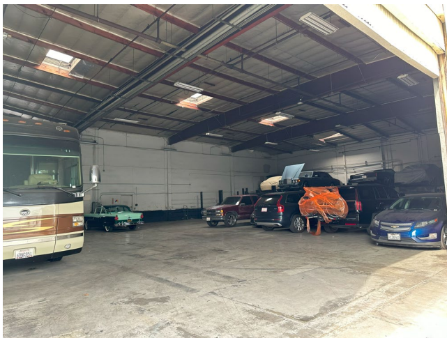
Westerly Bldg interior, showing skylights, view NW
