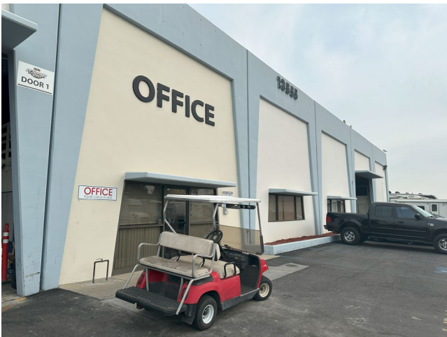
Easterly Bldg façade entry & fenestration, view NE
