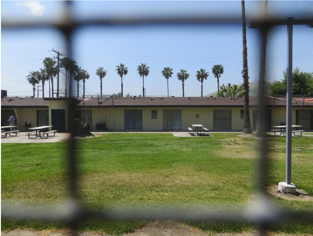
Photograph 7: South-facing view into the existing Shandin Hills Behavioral Health Center. For the biological field survey it was not necessary to go inside the interior, fenced facility.
