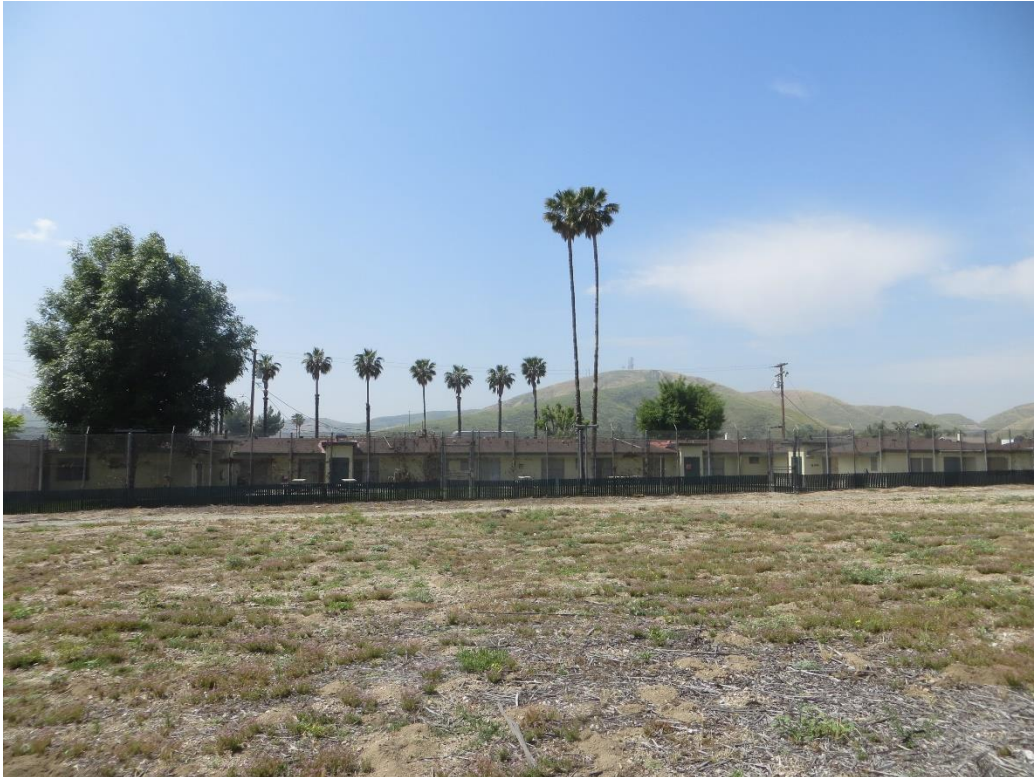
Photograph 2: South-facing view of the existing Shandin Hills Behavioral Health Center. These buildings are not part of the proposed construction.
