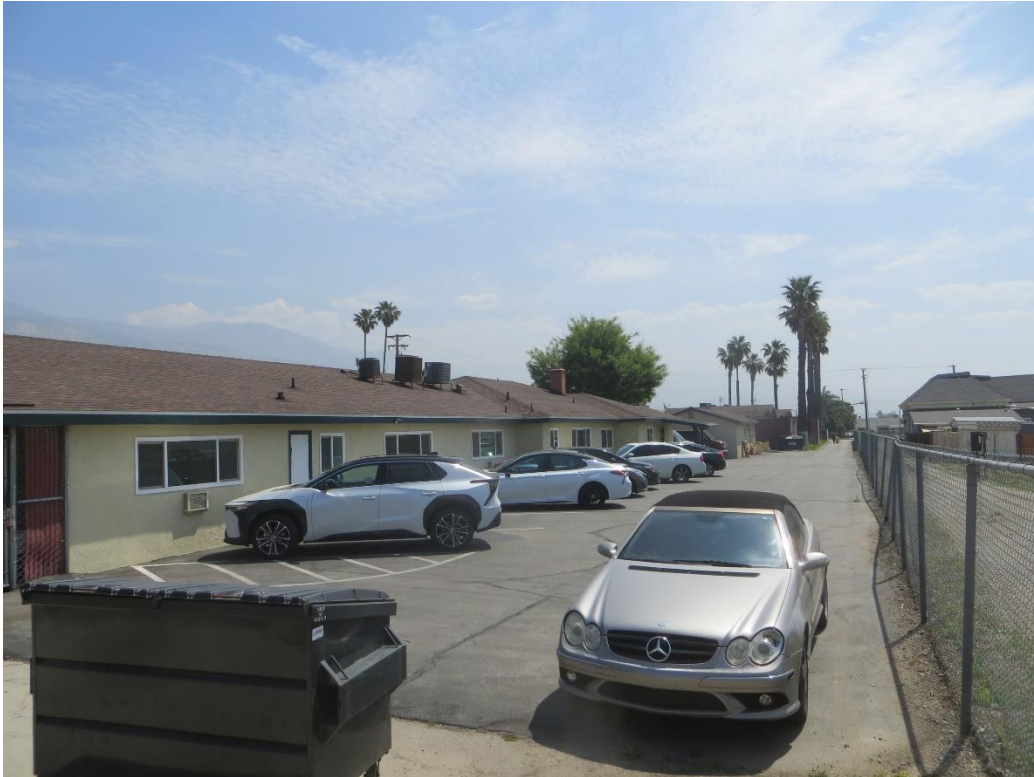
Photograph 6: Administrative buildings and offices located along the southeastern boundary of the project site. These buildings are proposed to be removed and replaced.
