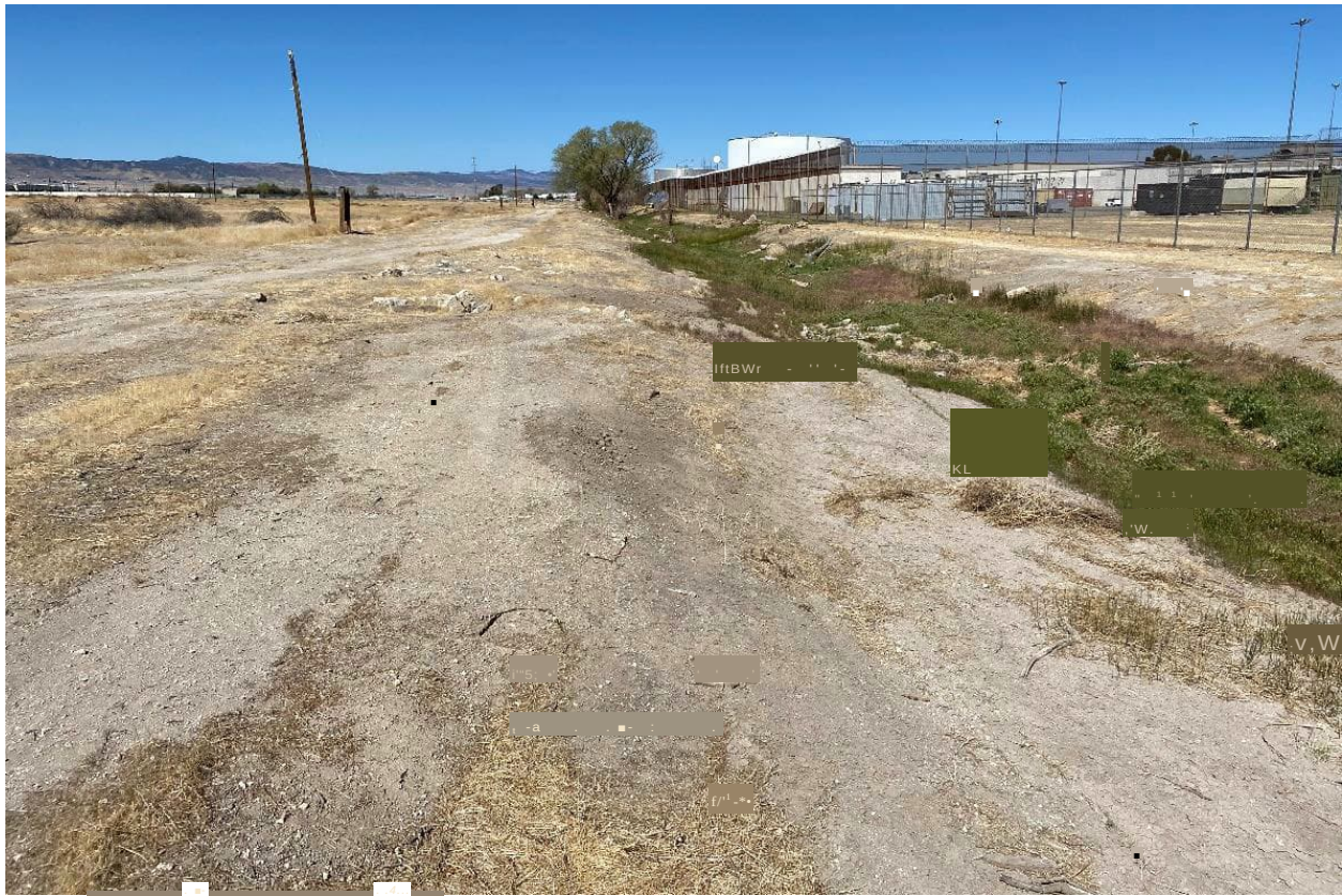
Photograph 9. West view (upstream) of drainage C within Study Area.
