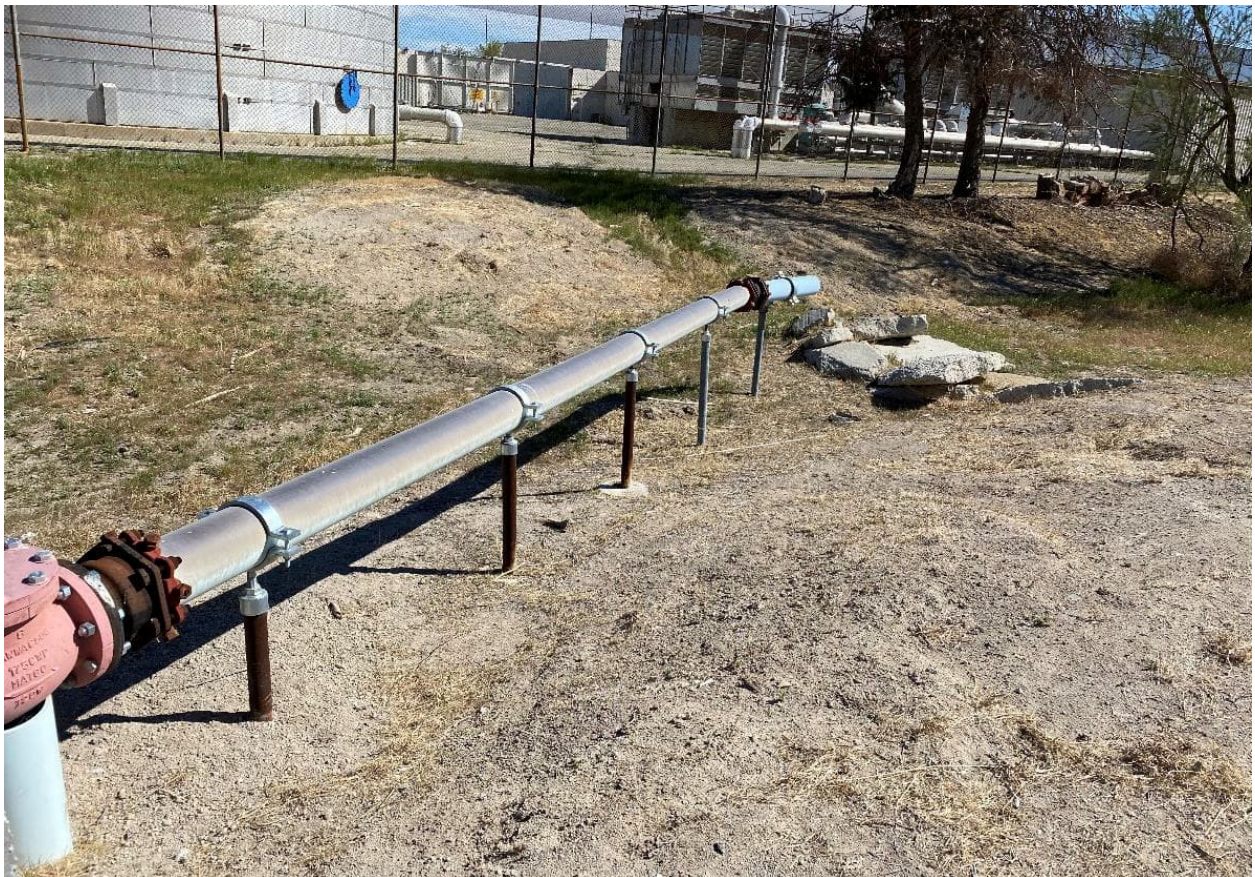
Photograph 6. Northeast view of drainage pipe leading to drainage C within Study Area.
