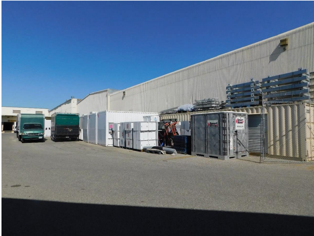
Exhibit 4. The west façade of the south part of the building mostly built by 1960 with additions done between 1980 and 1982, view facing north
