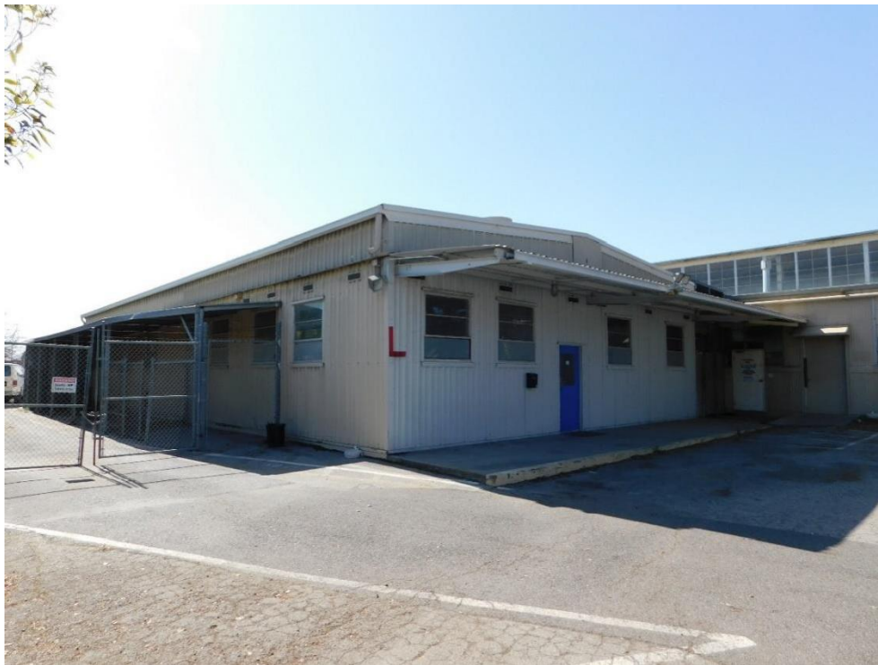
Exhibit 5. Auxiliary building L constructed between 1960 and 1965
