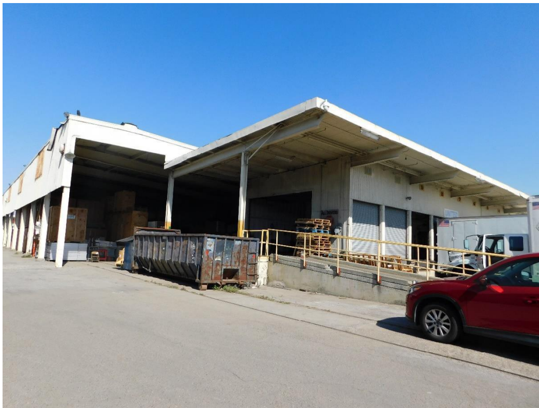
Exhibit 3. The south and west elevations of the structure that were present by 1948, view facing north
