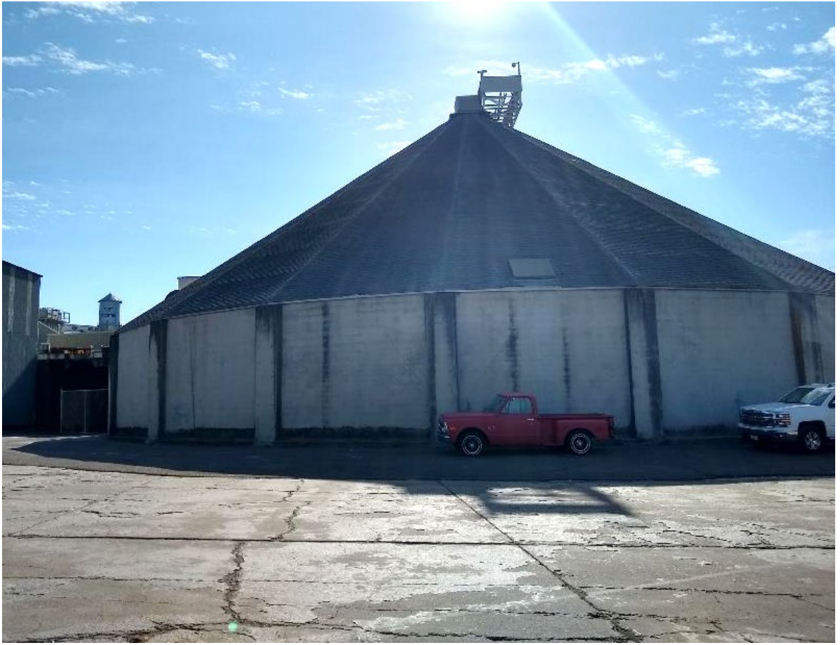
Photograph 4 Existing Cementitious Material Storage Bunker
