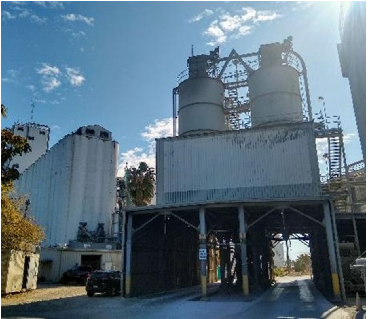
Photograph 6 Existing Truck Loading Station
