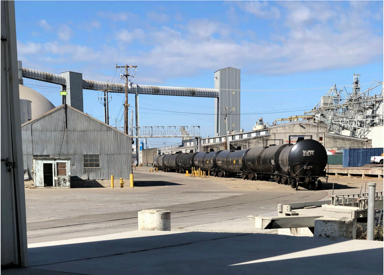
Photograph 7 Miscellaneous Building and Rail Operations
