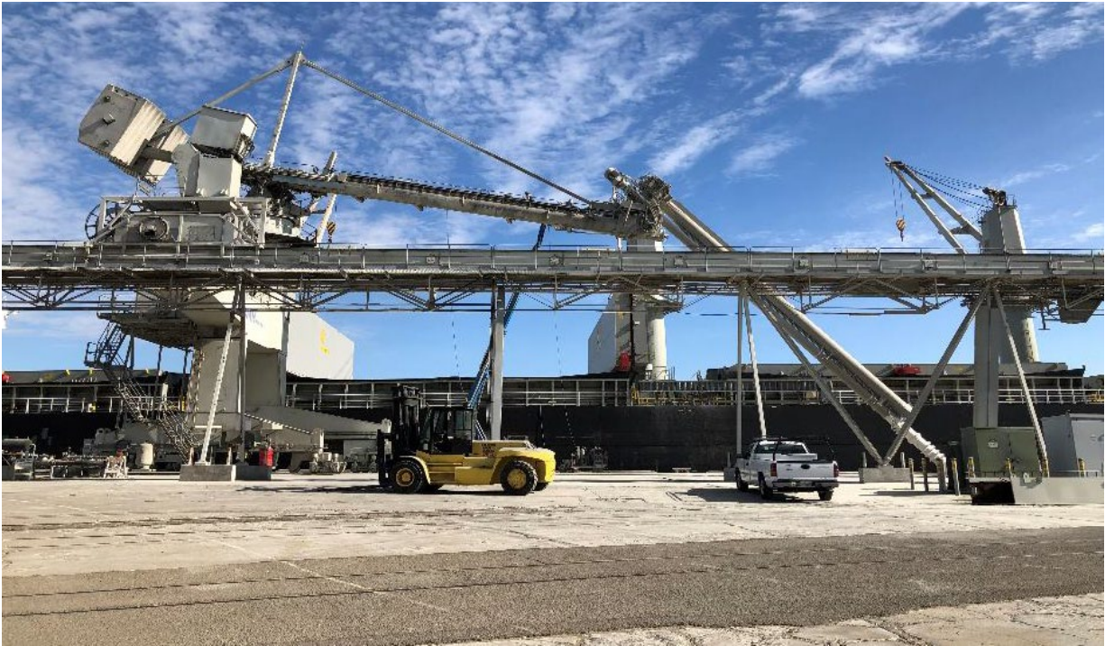
Photograph 2 Existing Ship Unloader
