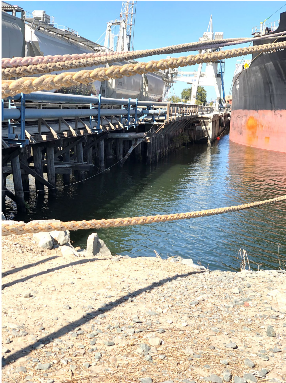
Photograph 1 Existing Berth 2 Dock Structure
