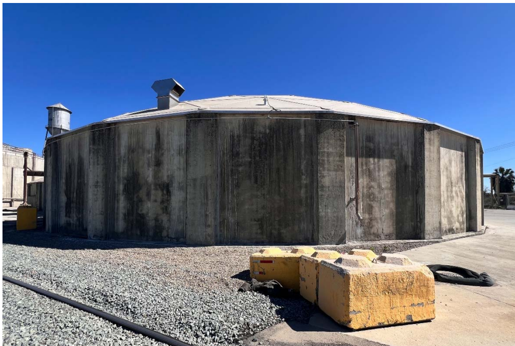
Bunker 4, View Northeast; Date: 3/13/2026
