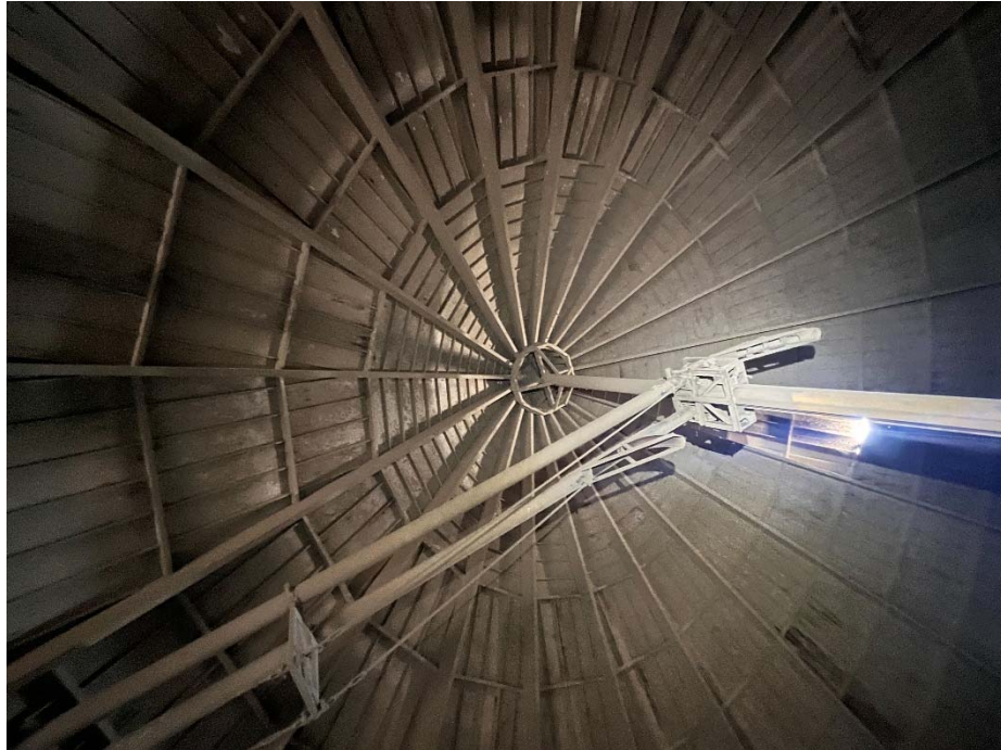
Bunker 5 Interior; Date: 3/13/2026
