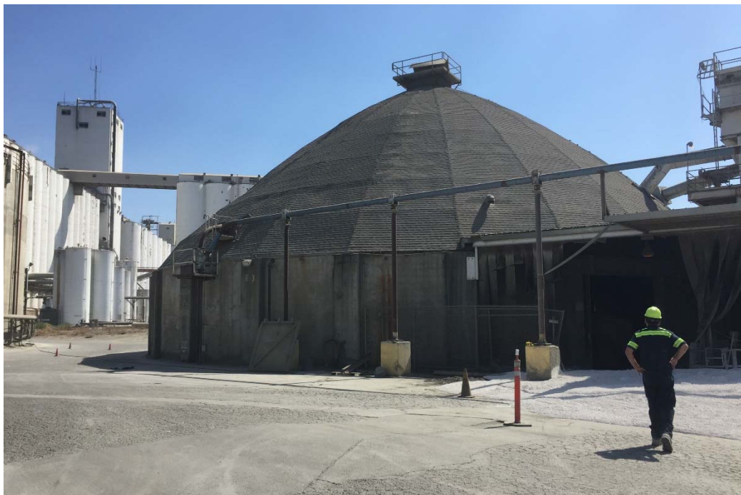
Bunker 3, View Southeast; Date: 2019
