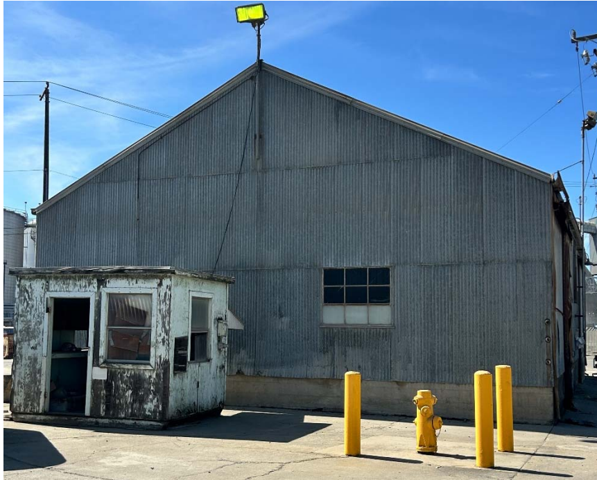
East Elevation, View Southwest; Date: 3/13/2026
