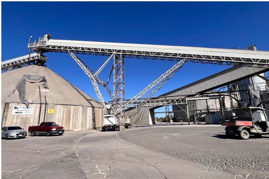
Bunker 5 (left) and Mobile Conveyor, View Northeast; Date: 3/13/2026
