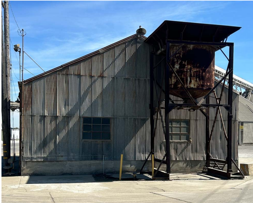
East Elevation, View West; Date: 3/13/2026
