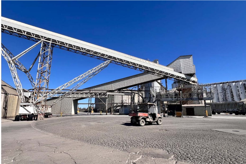
Mobile Conveyor and Conveyor Tower, View East; Date: 3/13/2026
