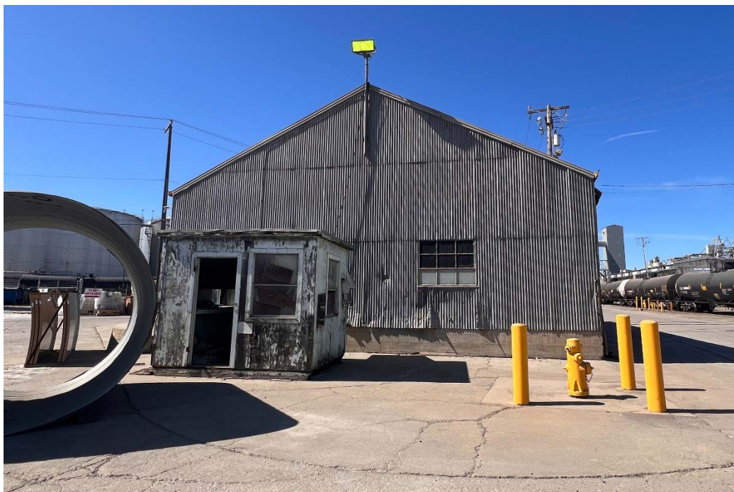
East Elevation, View West; Date: 3/13/2026
