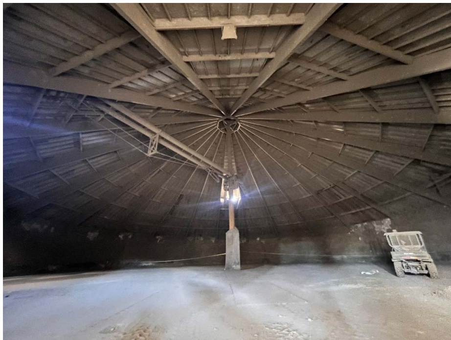
Bunker 5 Interior; Date: 3/13/2026
