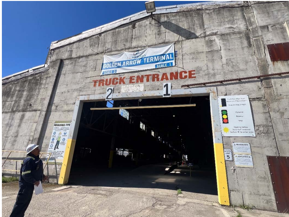
East Elevation, View Southwest; Date: 3/13/2026
