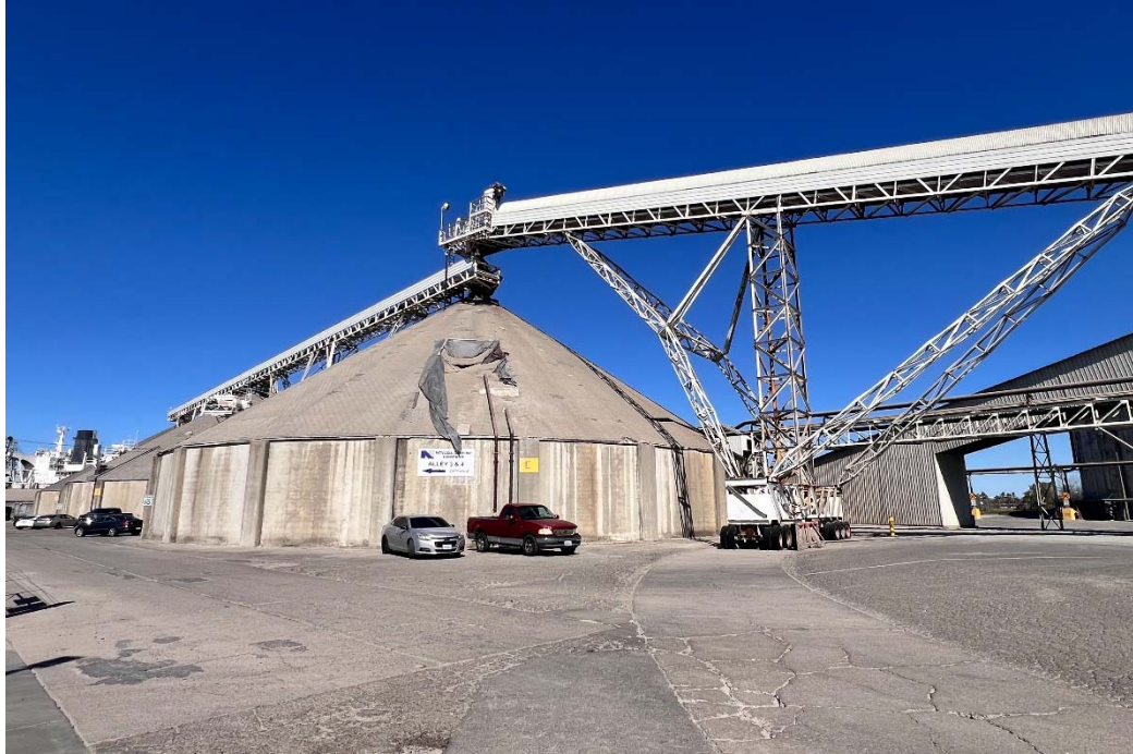
Bunkers 5 (foreground) 6, and 7; View North; Date: 3/13/2026
