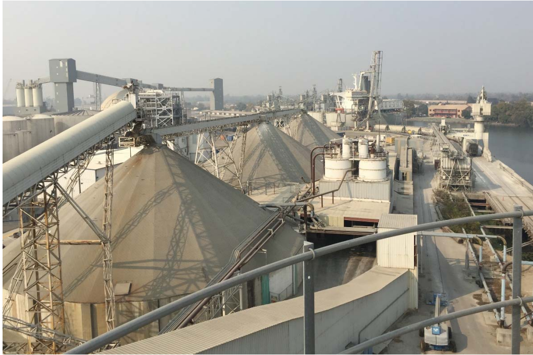
Bunkers 5, 6, and 7 from Conveyor Tower, View Northwest; Date: 2019
