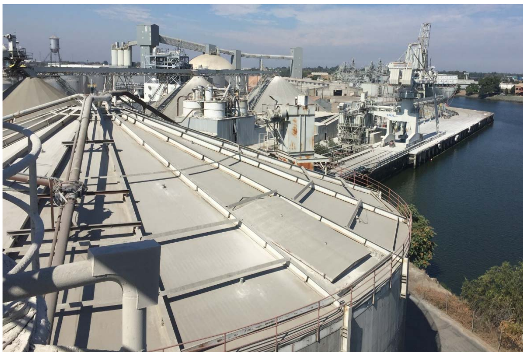
View of Bunker 1 (foreground) from Loading Station, View West; Date: 2019
