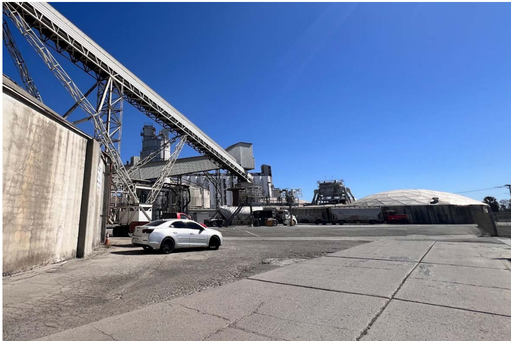
Bunker 5 (left) and Conveyor Tower (center; Bunker 4 on right), View Southeast; Date: 3/13/2026
