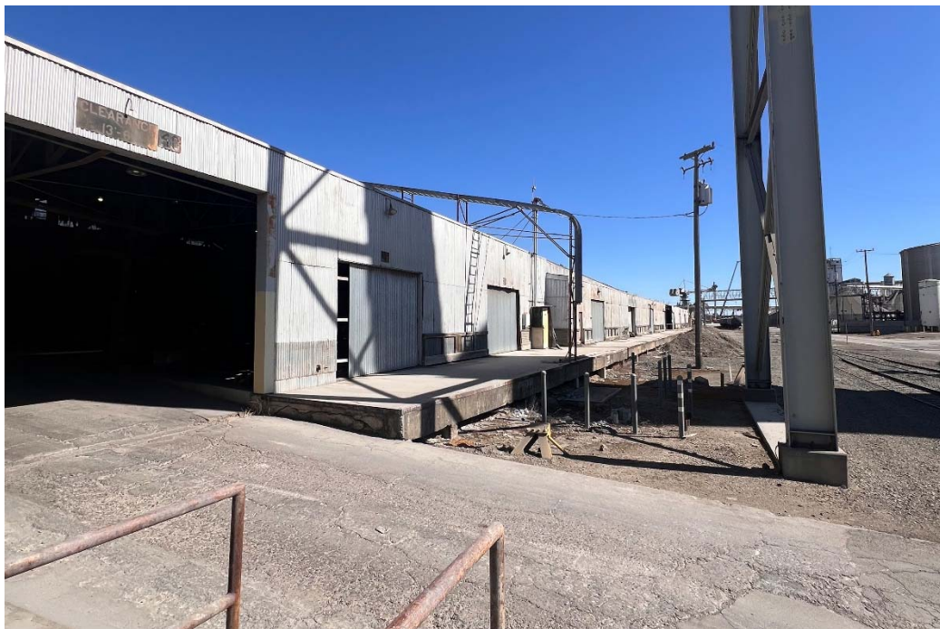
South Elevation, View Northeast; Date: 3/13/2026
