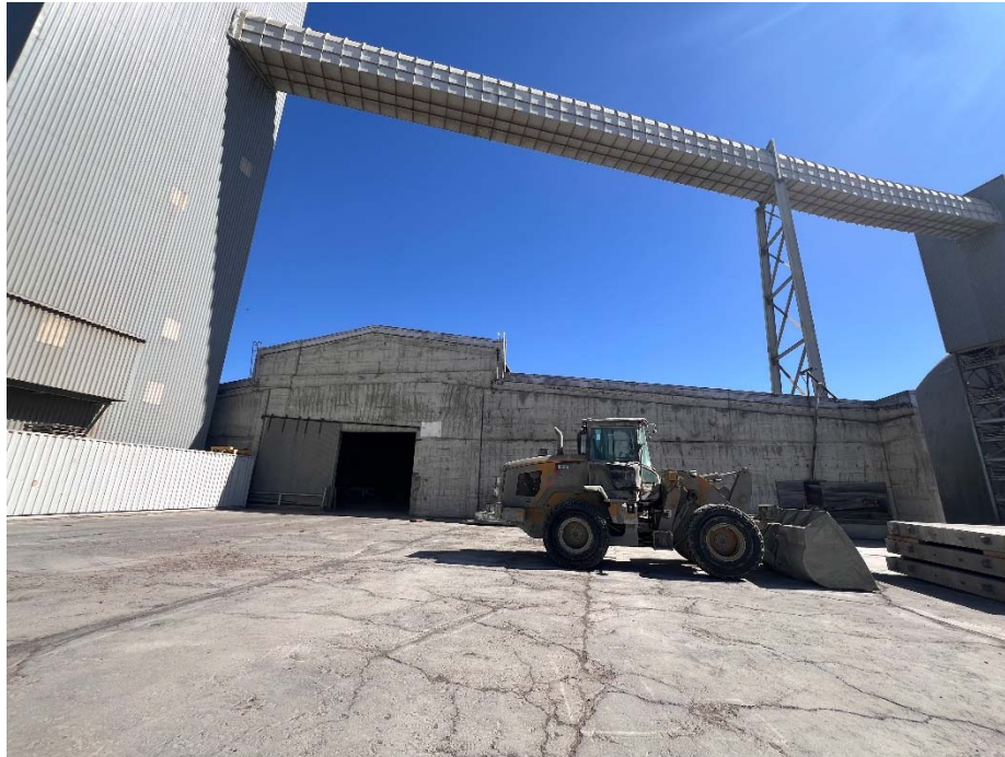
West Elevation, View East; Date: 3/13/2026
