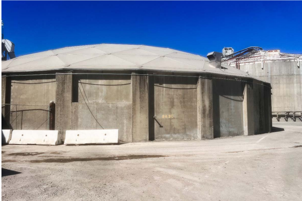
Bunker 3, View North; Date: 3/13/2026
