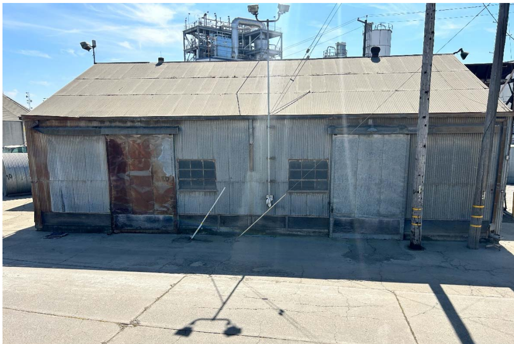
North Elevation, View South; Date: 3/13/2026
