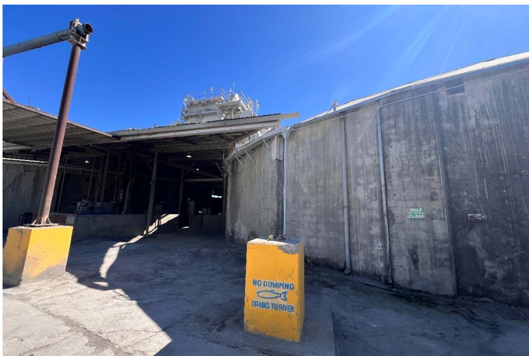
Bunker 4 and former Loading Station, View Southeast; Date: 3/13/2026
