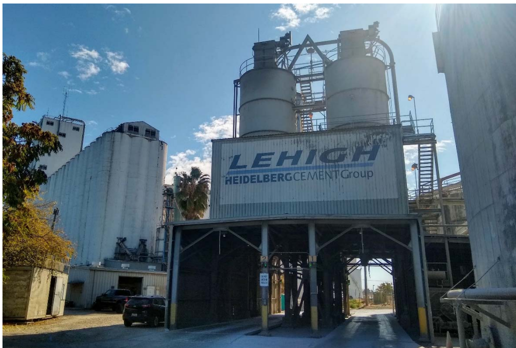
Truck Loading Station, View Southeast; Date: 3/13/2026
