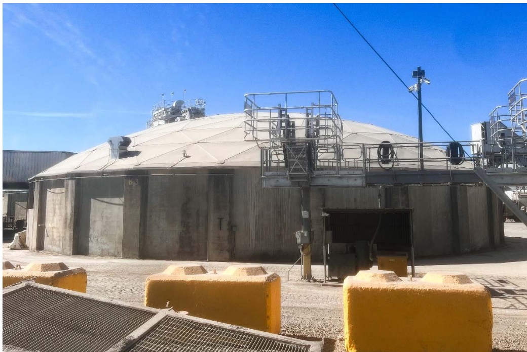
Bunker 3, View West; Date: 3/13/2026
