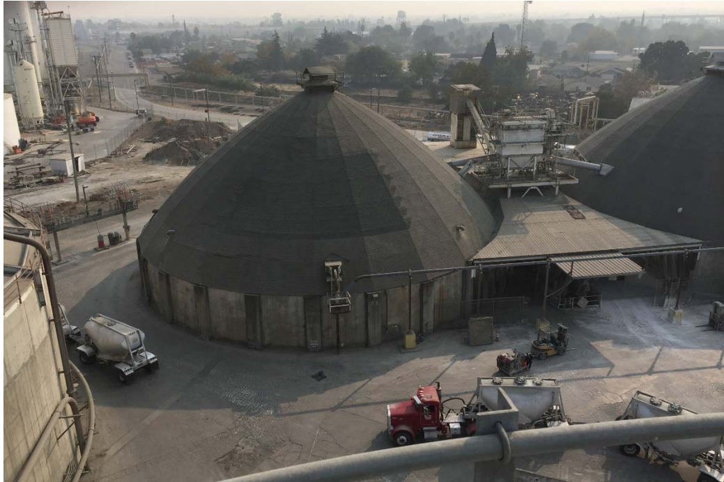
Bunkers 3 and 4, View Southeast; Date: 2019
