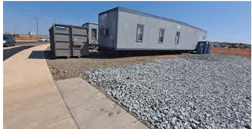
Looking north at temporary construction trailers on the western portion of the site.
