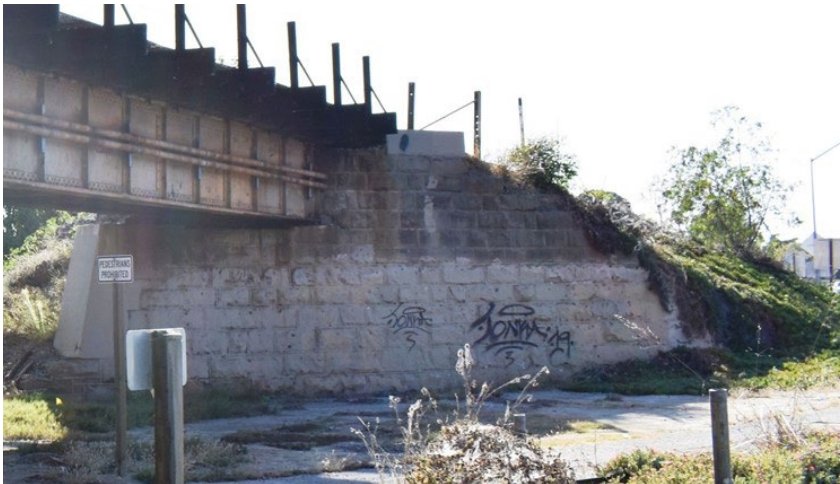
Photograph 3. Western sandstone abutment, looking west
