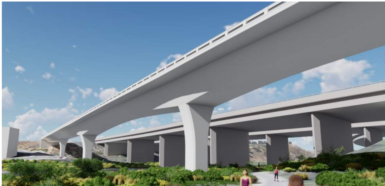
FIGURE 4: Haunched Box Girder Type Bridge - Computer Rendering
