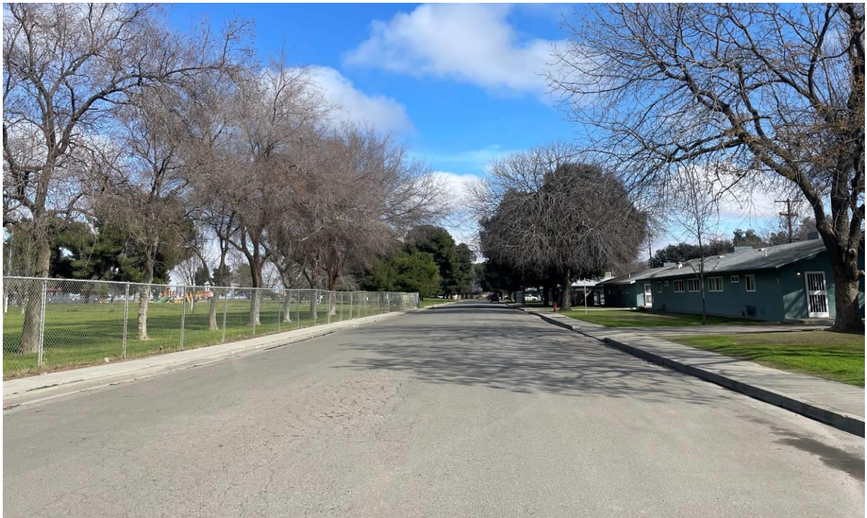
Photo 2: Another representative photo of a paved street within one of the sewer main work areas.
