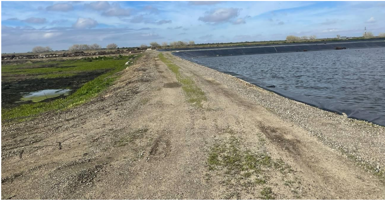
Photo 7: Representative photo of the project site's WWTP work area and adjacent land use. Work area is to the left of the full treatment pond.
