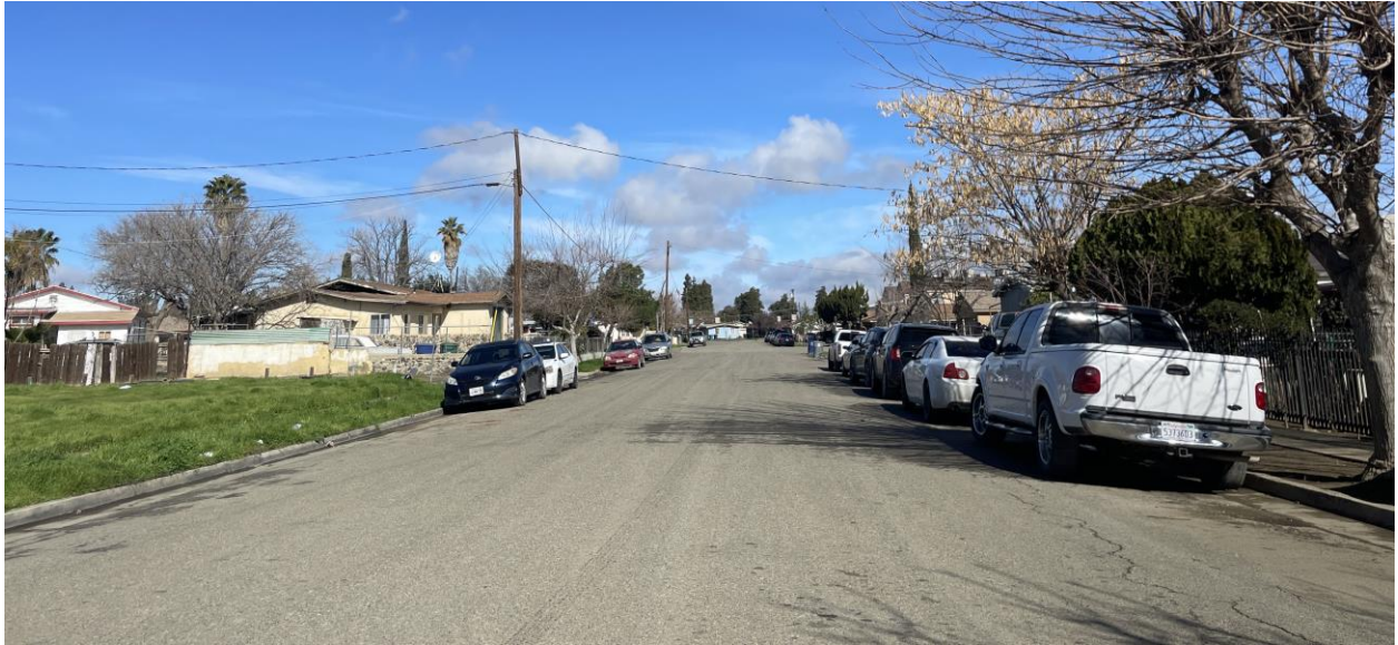
Photo 1: Representative photo of a paved street within one of the sewer main work areas. Trees and a green space are immediately outside work area boundaries.
