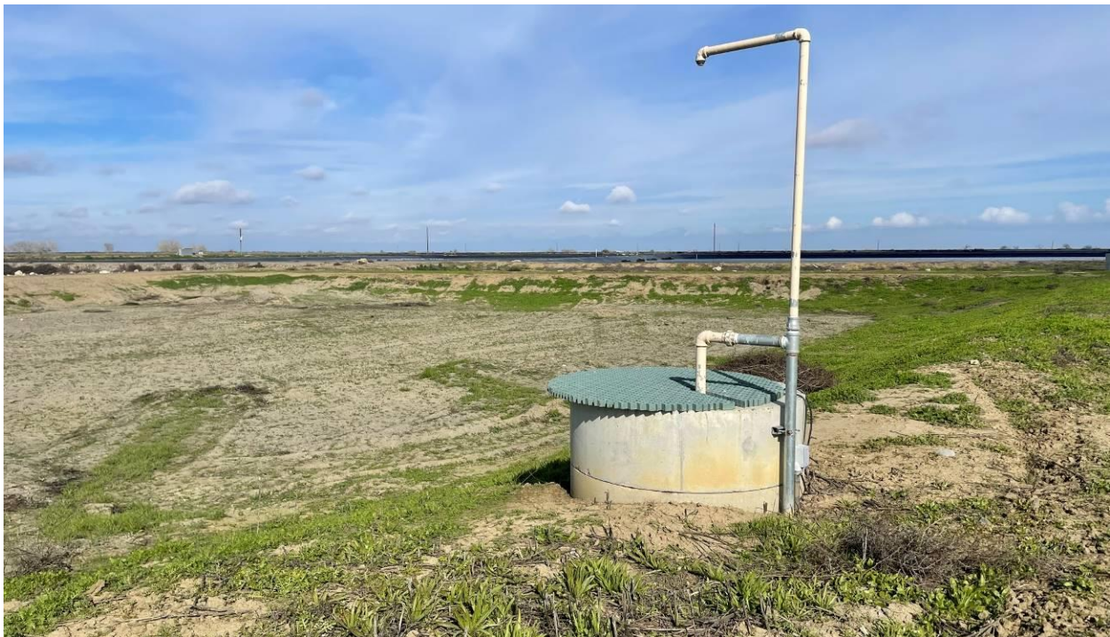
Photo 8: Dry wastewater treatment pond with some established vegetation.
