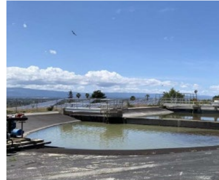
Sludge holding basins
